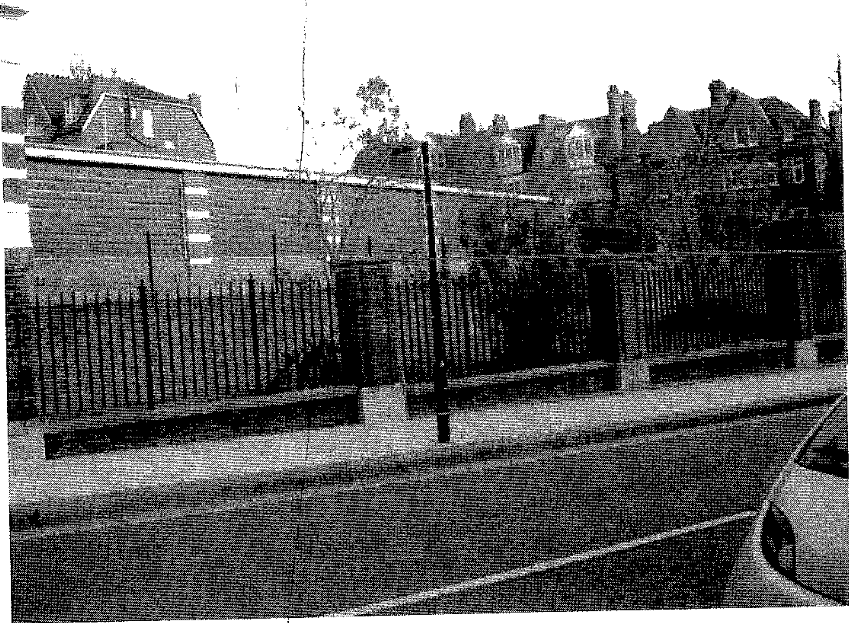
Photo of Part of Boundray Wall to be Temporarily Removed
