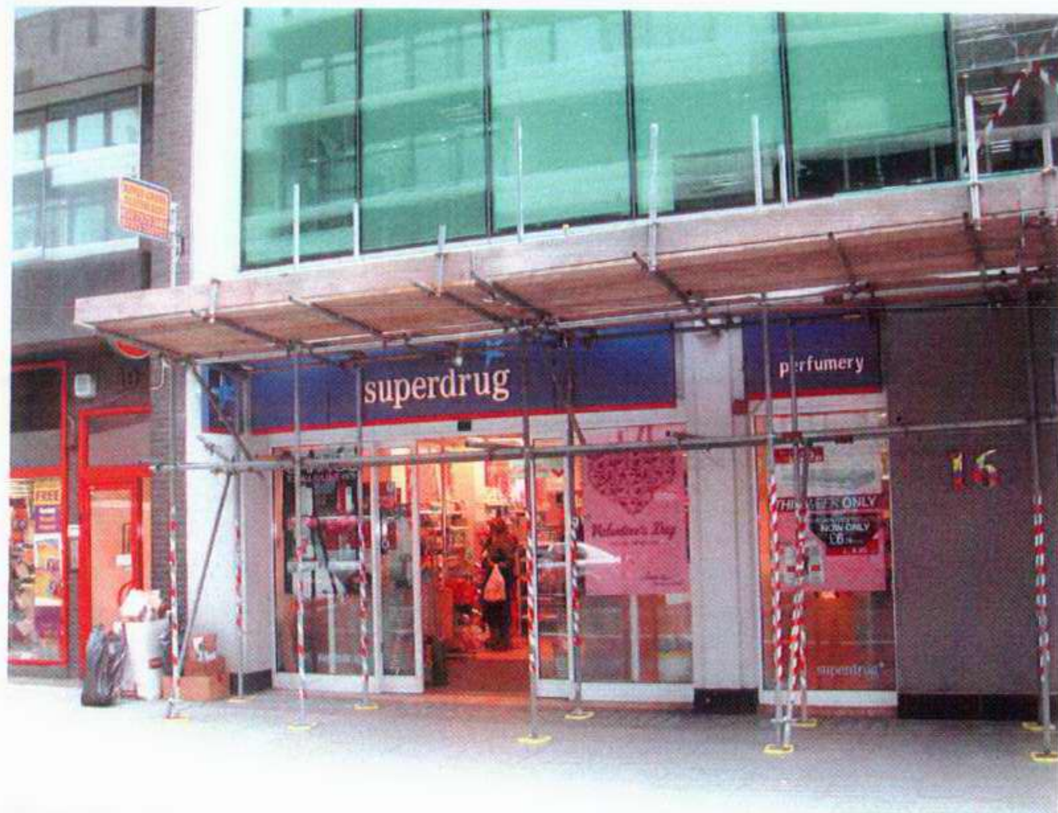
Existing Site Photograph
