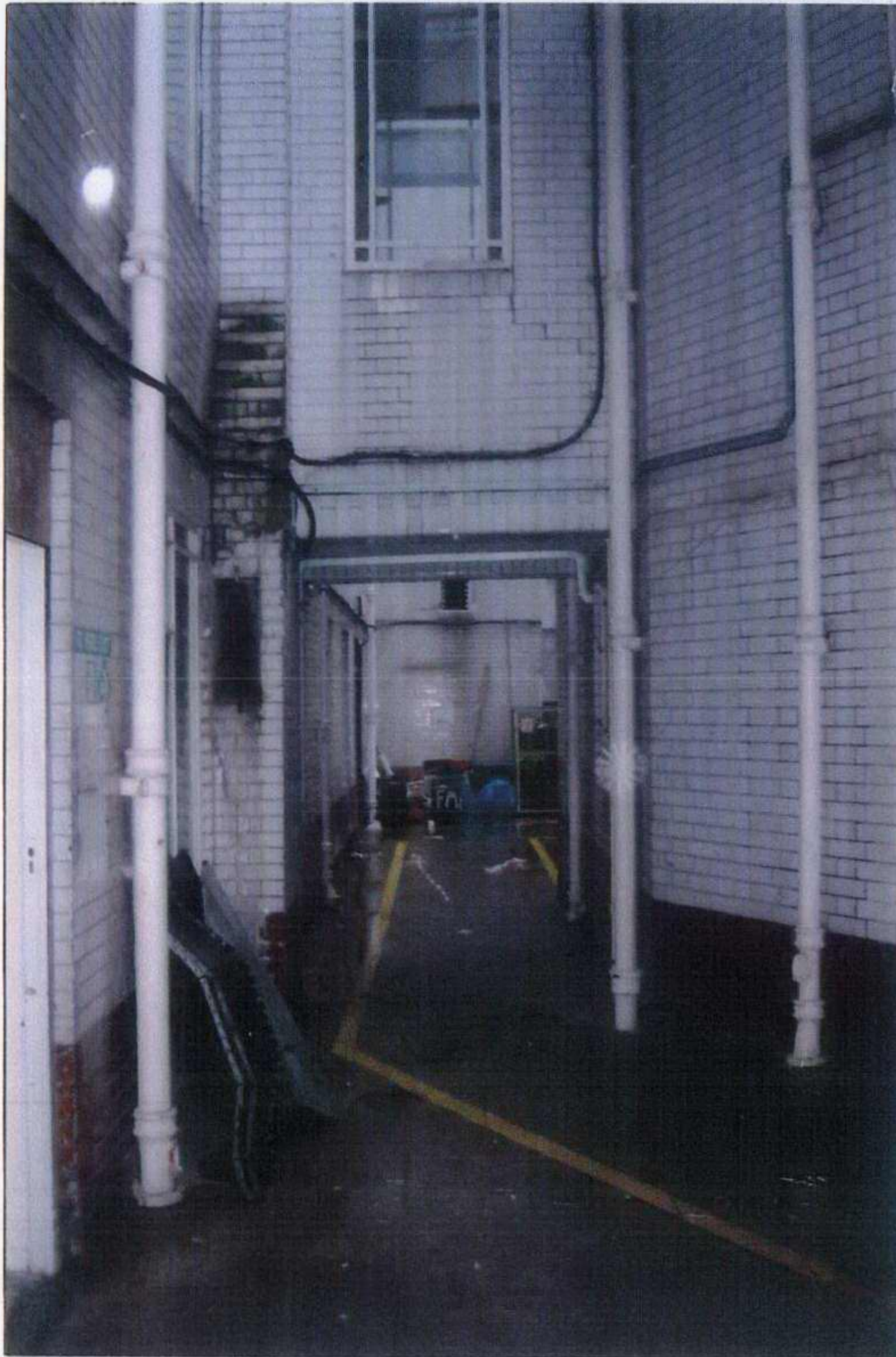
View from North Courtyard
