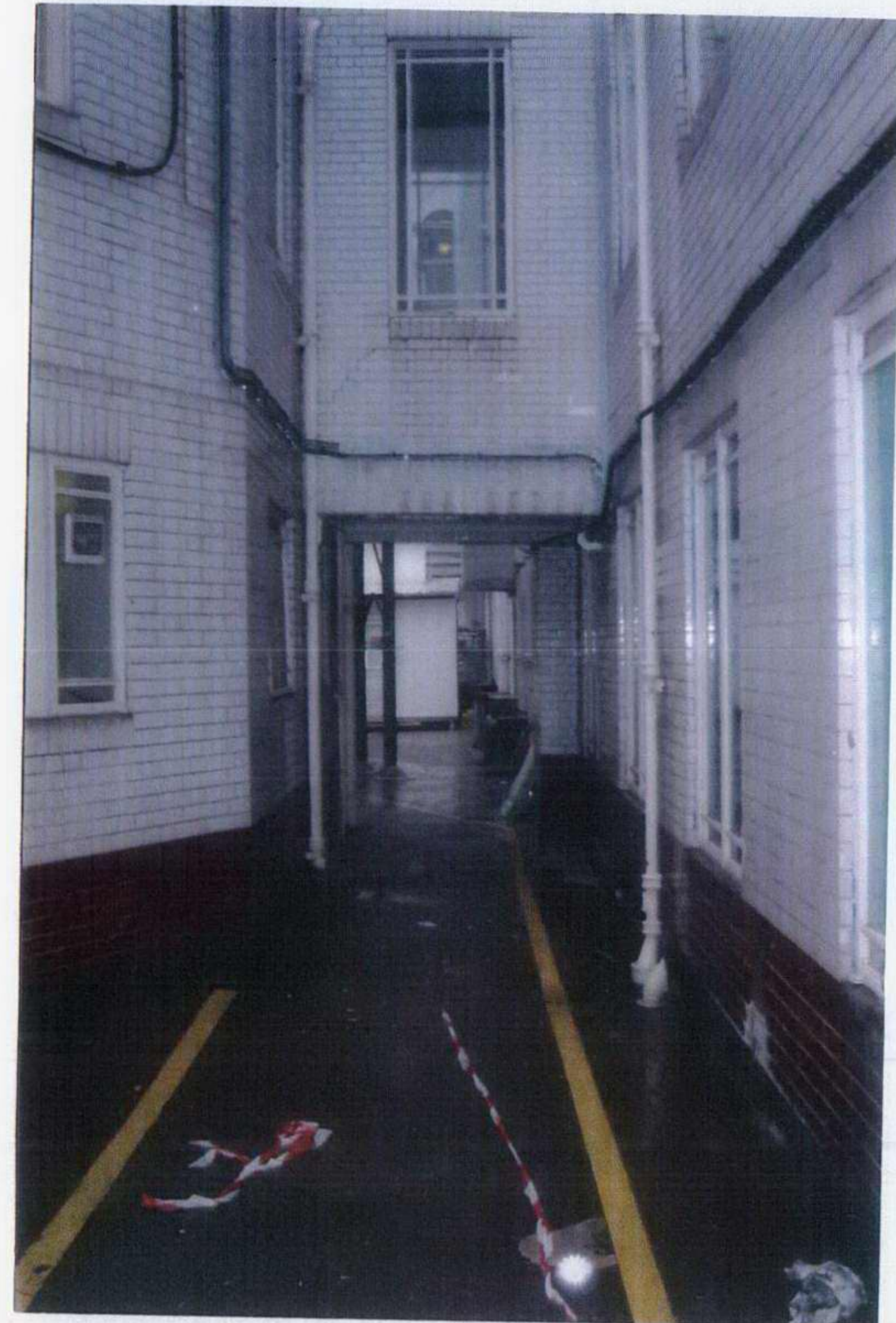
View from South Courtyard
