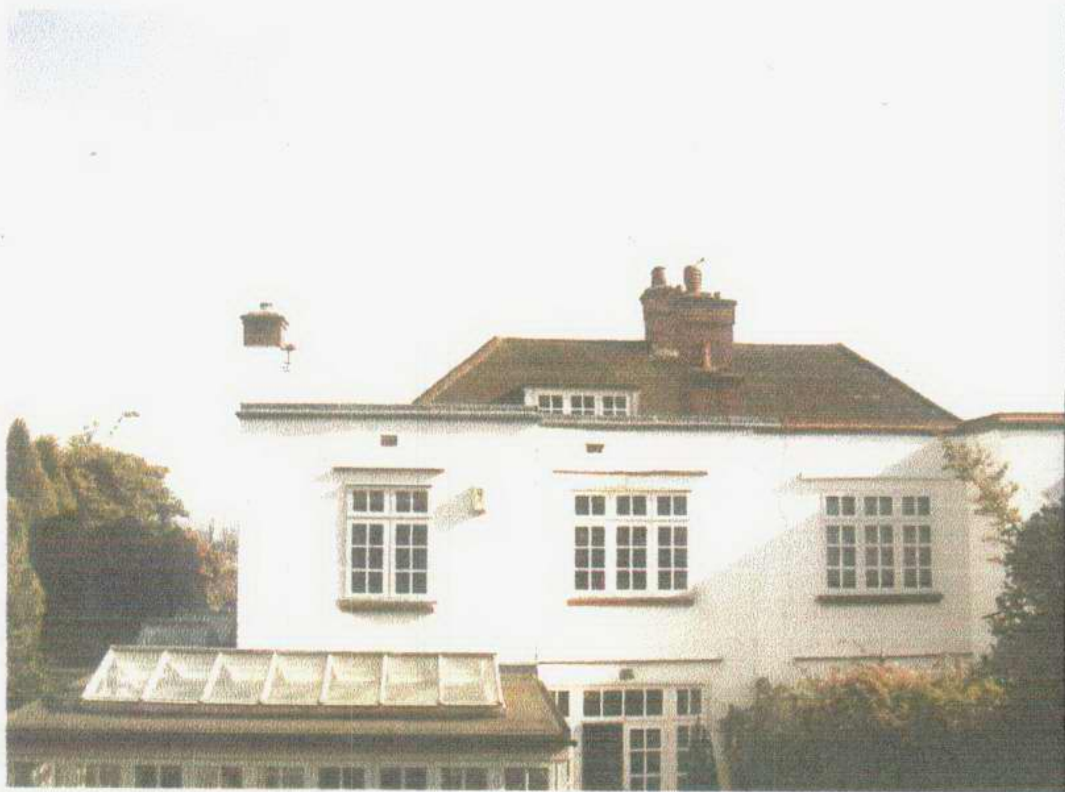
VIEW FROM REAR ELEVATED.
