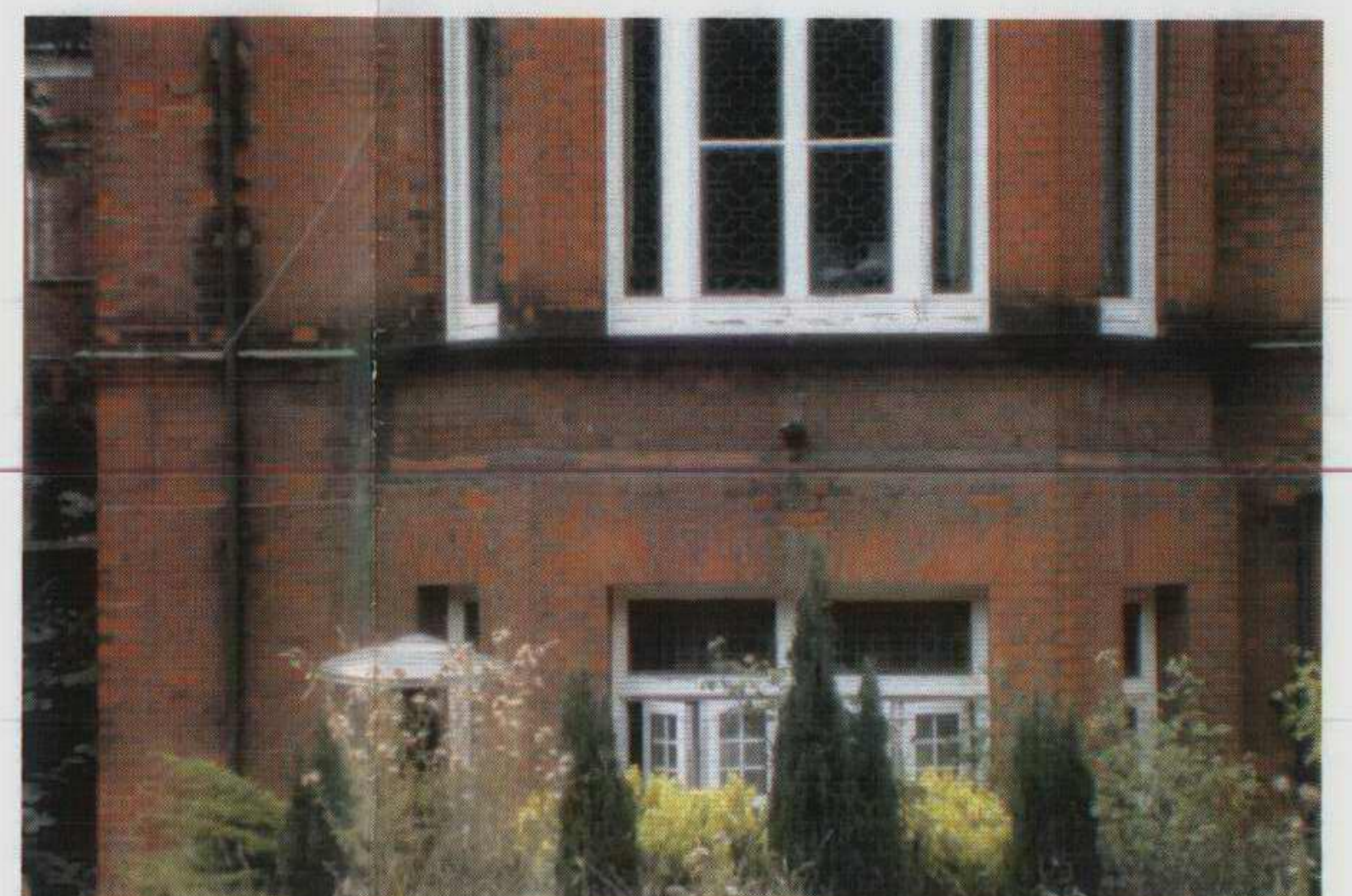
62 Eton Avenue - Existing Building Photographs - 1
