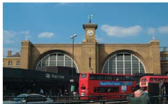
Euston Road frontage of King's Cross Station
