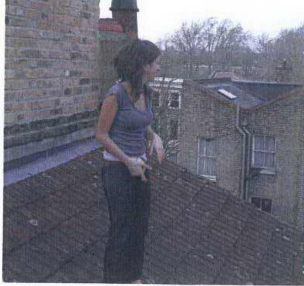
Existing valley roof to No. 47
