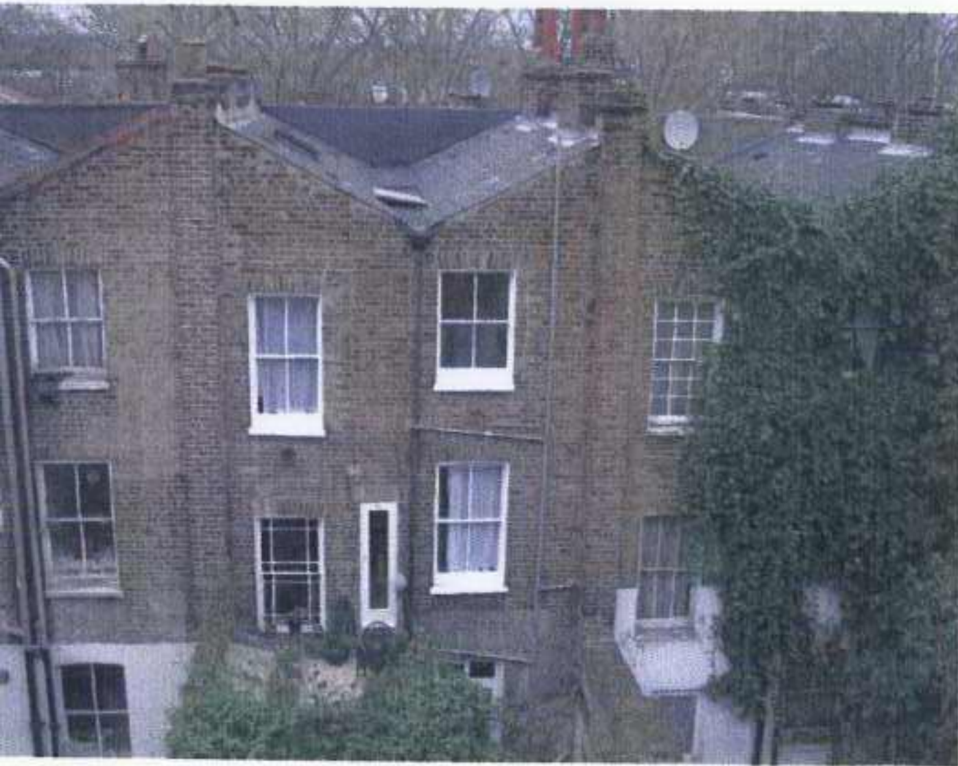
View from No. 47 showing rear of terraces properties on St Martins Close
