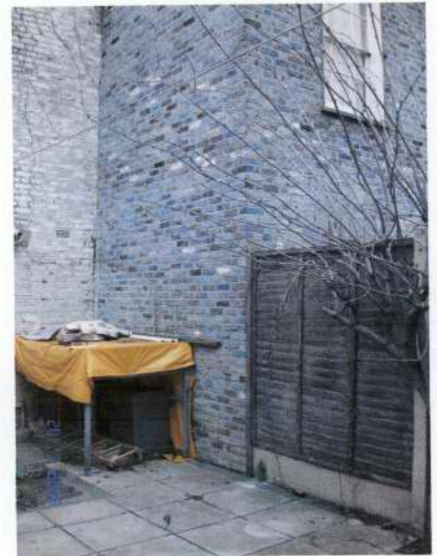
LOOKING TOWARDS REAR ELEVATION OF NO 18
