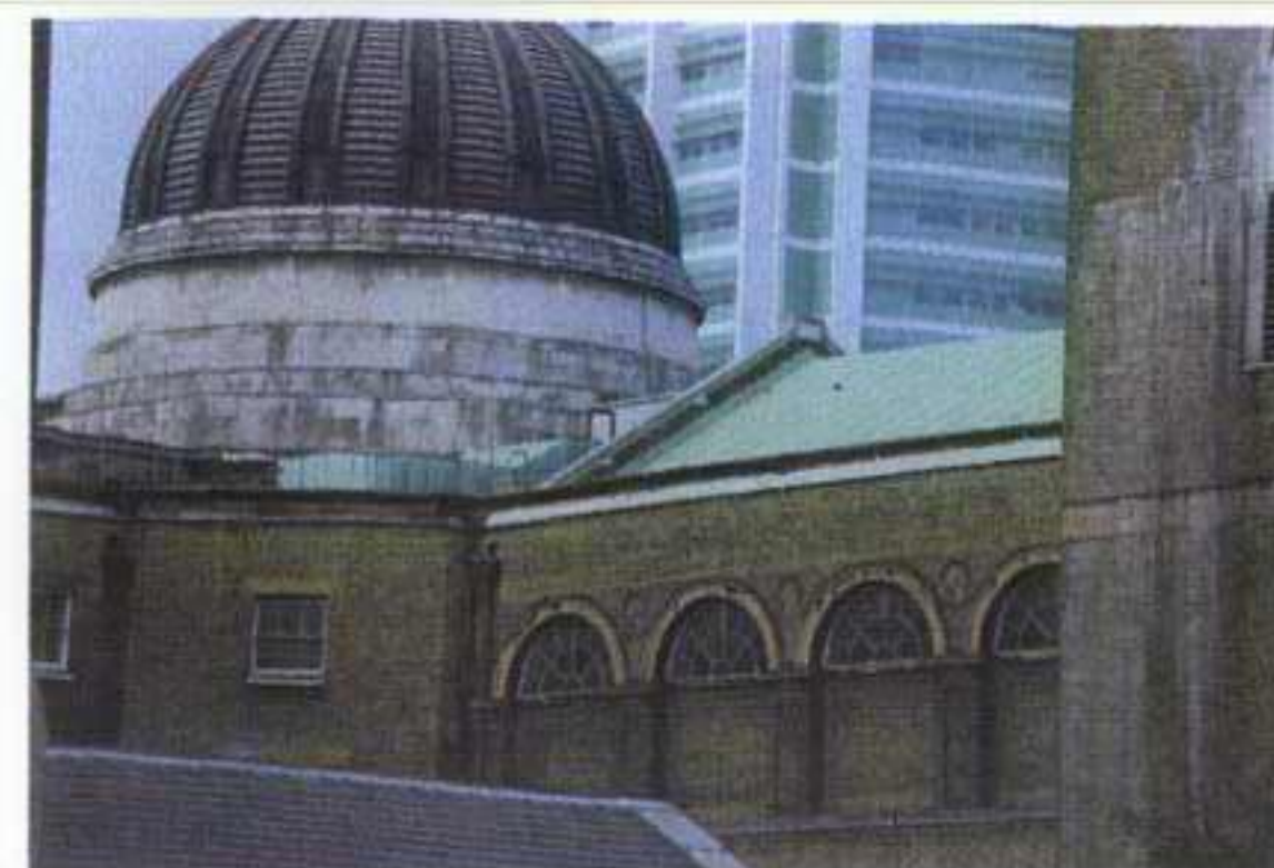
Figure 8 Views of the main University Building showing the extensive use of copper as a roofing material.
