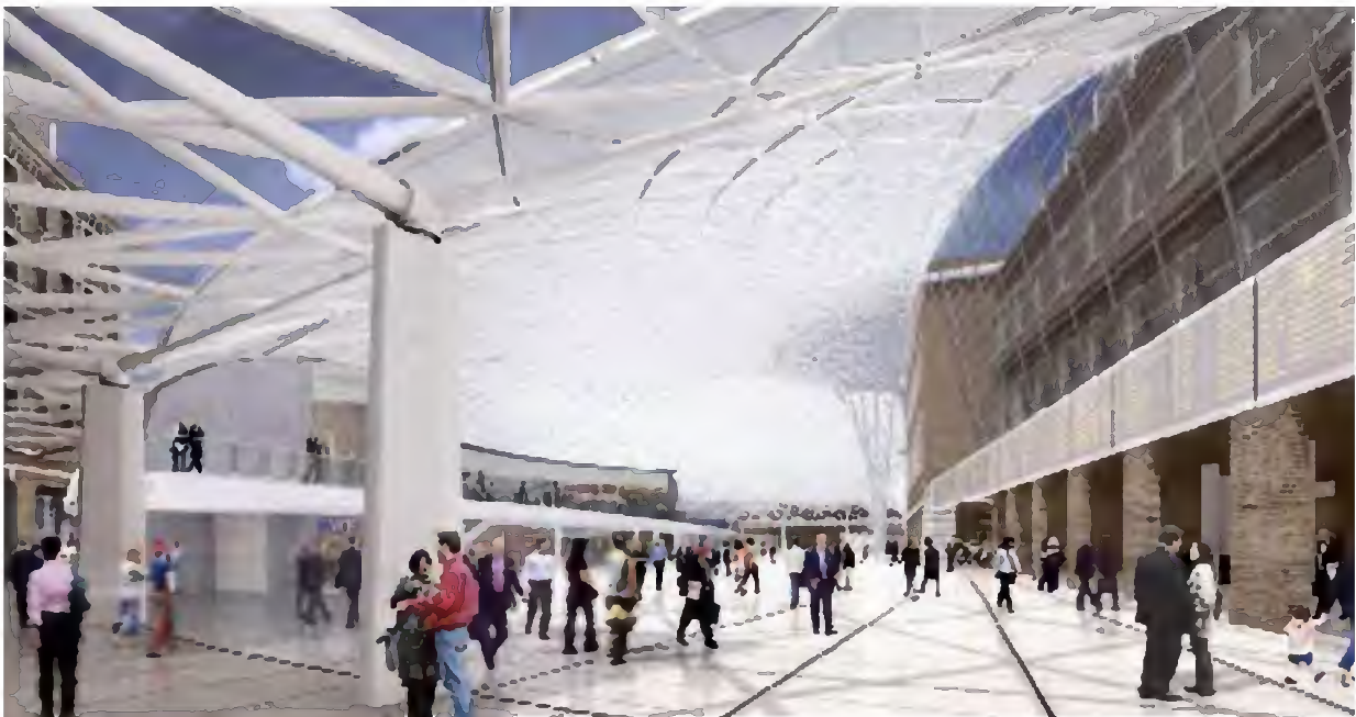
New Western Concourse Roof, naturally ventilated throughout.
