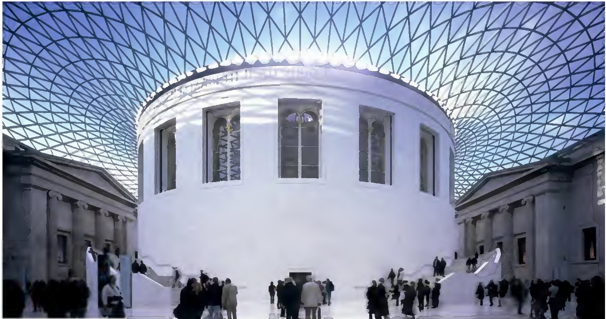
British Museum, Great Court, displacement ventilation and mechanical extract is required to control the environment.
