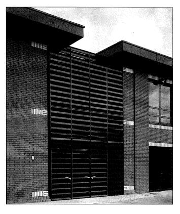
EMTEC LAAC 15 and LAAC 30 Acoustic Louvres can be installed as individual units or by bolting more than one unit together openings of any size can be accommodated. Each louvre has a robust outer framework which acts as vertical or horizontal mullions when several units are fixed together. If a continuous blade effect is preferred this can also be supplied.
