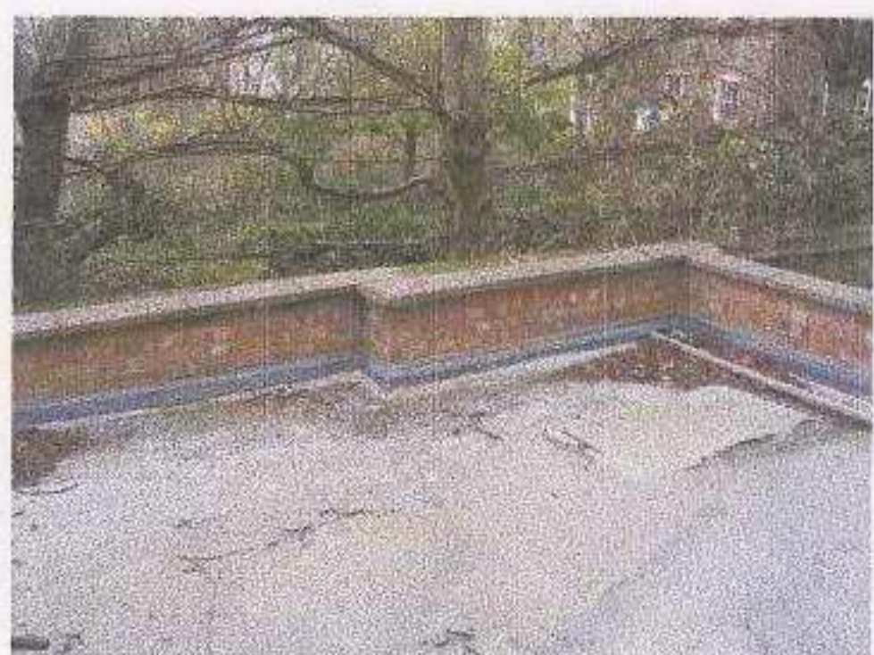
View of Flat roof
