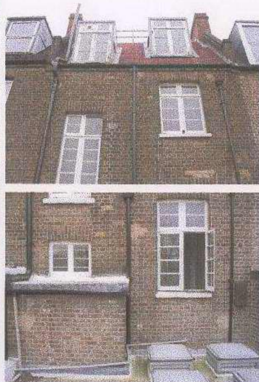
View of back of 9 Heath street
