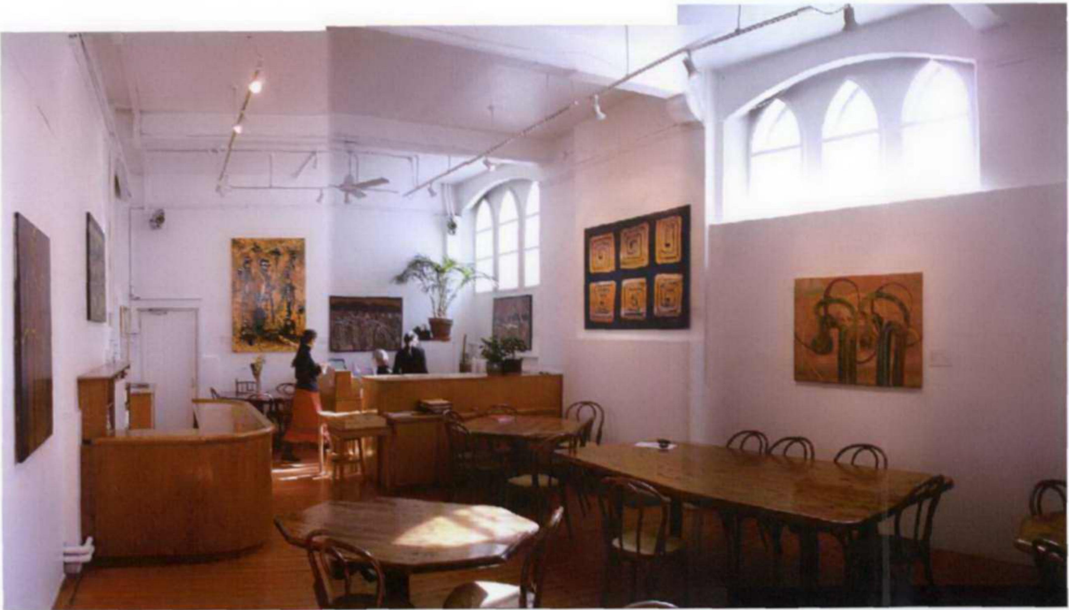
EXISTING INTERIOR VIEW TOWARD CHIMNEY BREAST
