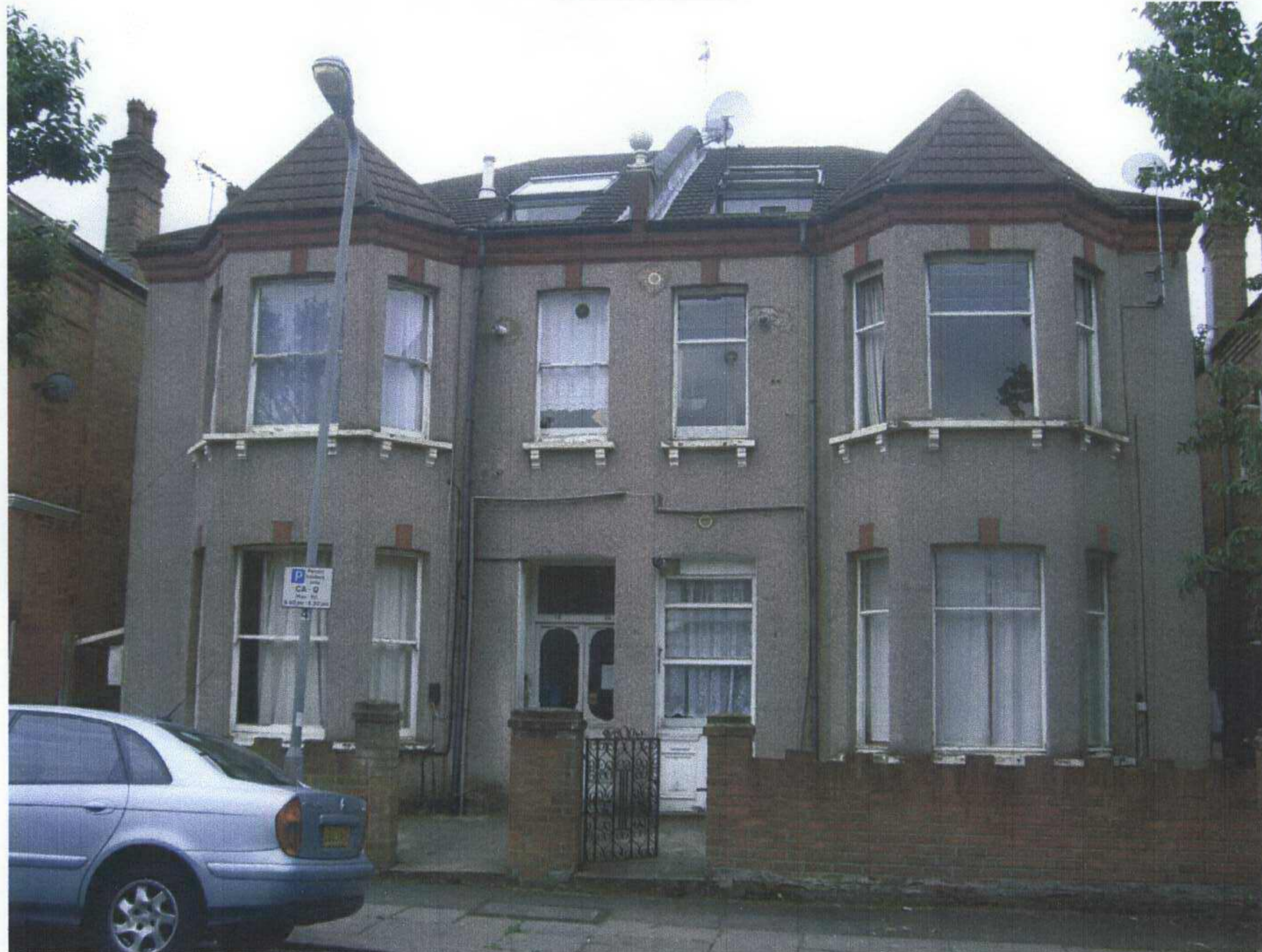
Front Elevation of 13-15 Skardu Road 6887/PH01
