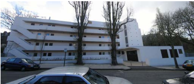
Isokon Flats- Once said to be the ugliest building in Hampstead, now Grade 1 listed and recently restored.
