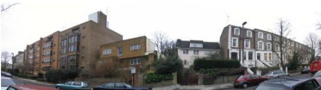
Local streetscape in winter- note disparity in scale, exposure of blank party walls.
