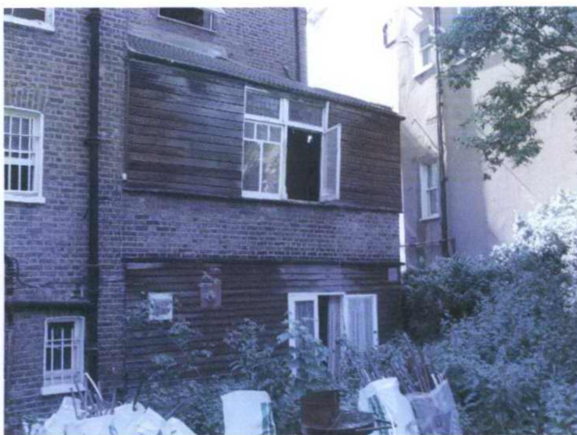
Part Rear Elevation looking SW.
