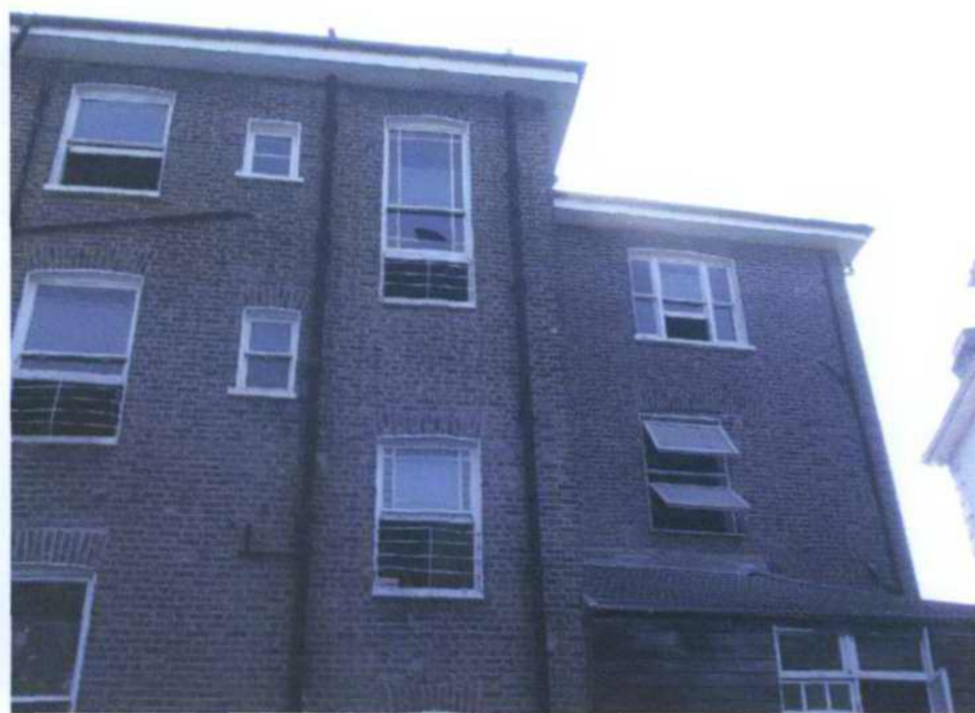
Part Rear Elevation looking S.
