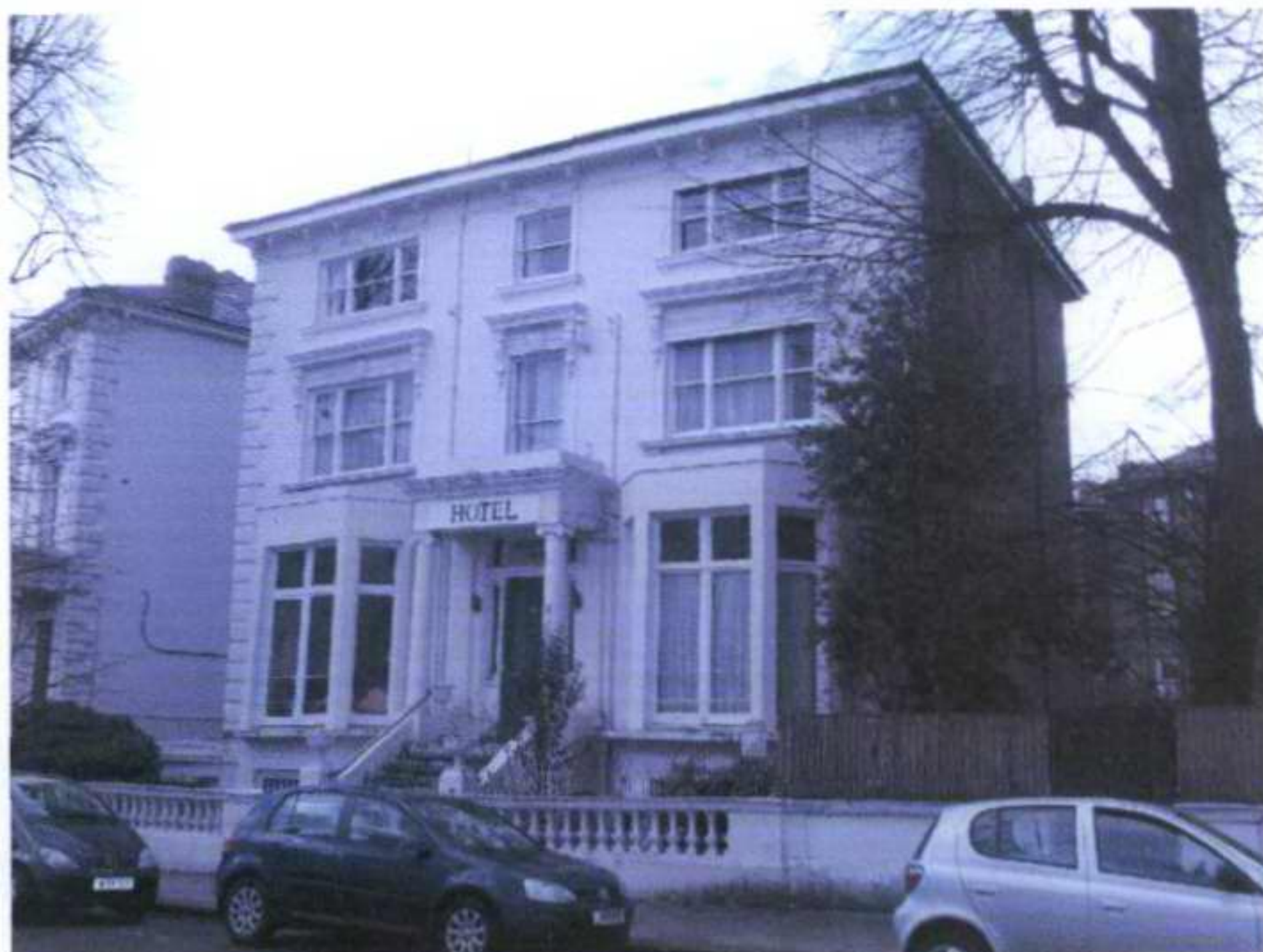
Front Elevation looking NW.
