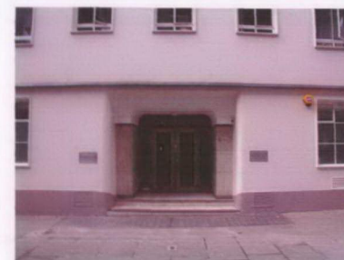
General view of the entrance requiring a shutter
