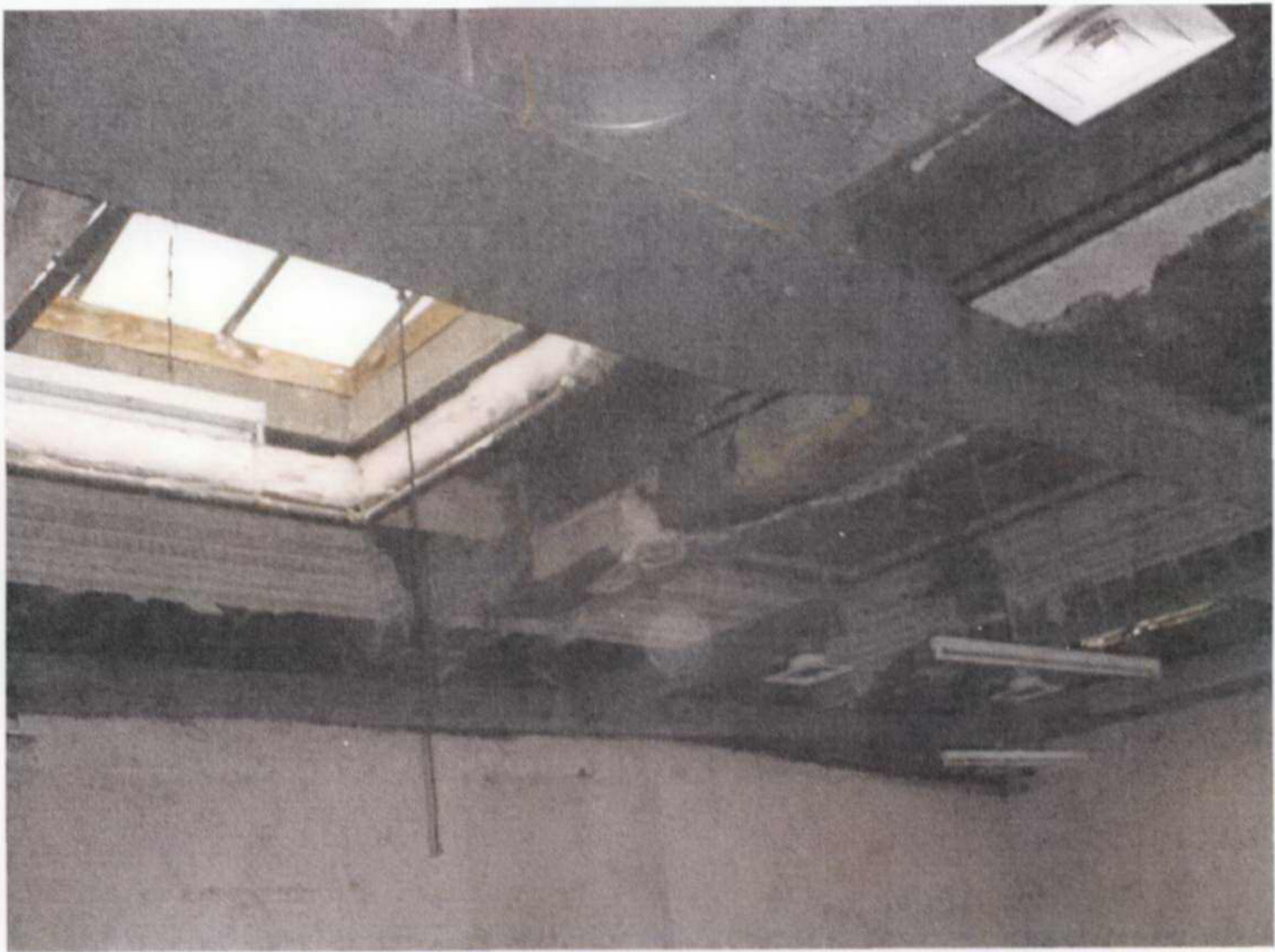
Ref: 005 – View on Roof Light and Ductwork
