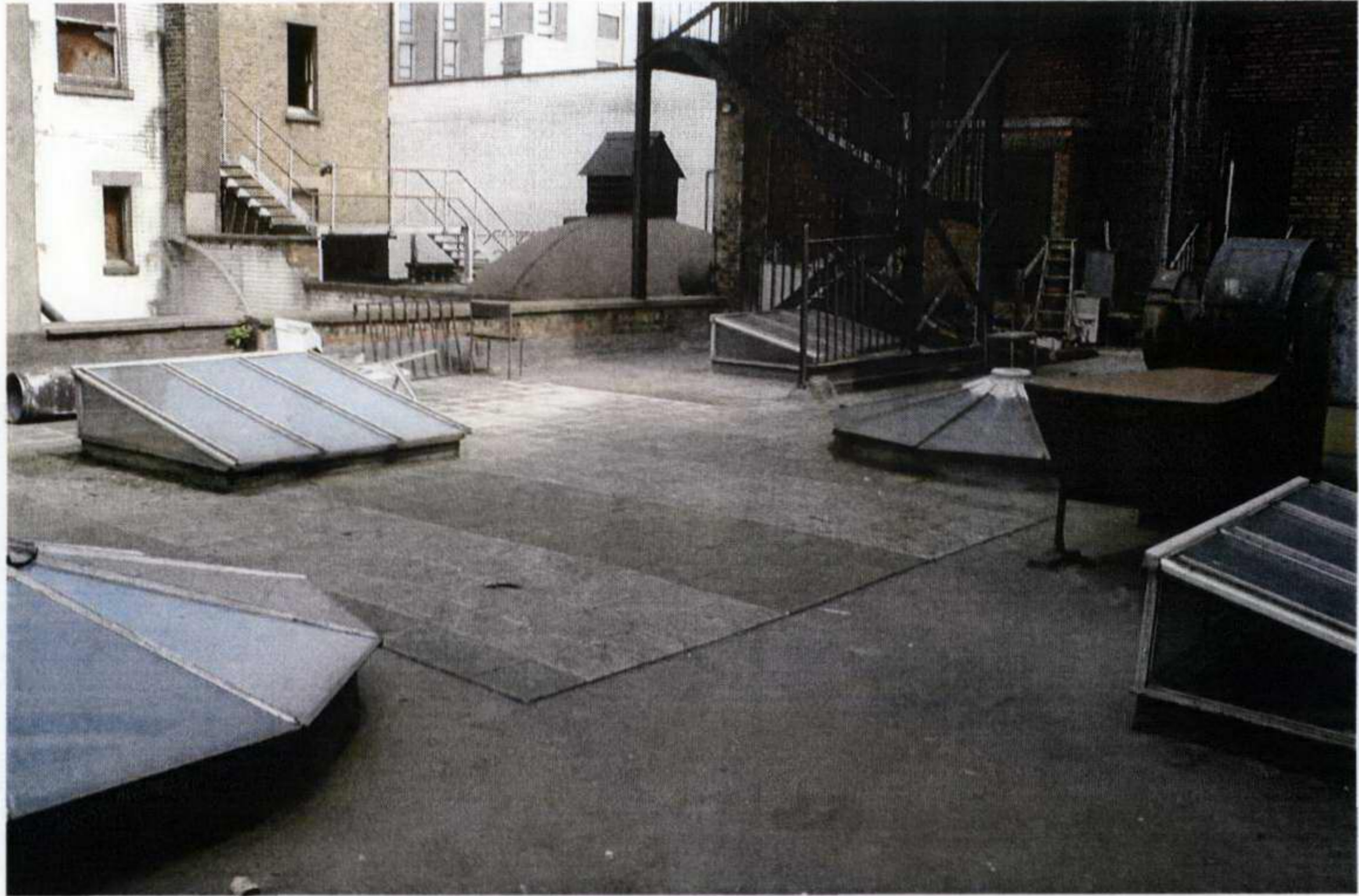
Ref: 003 – General Roof View
