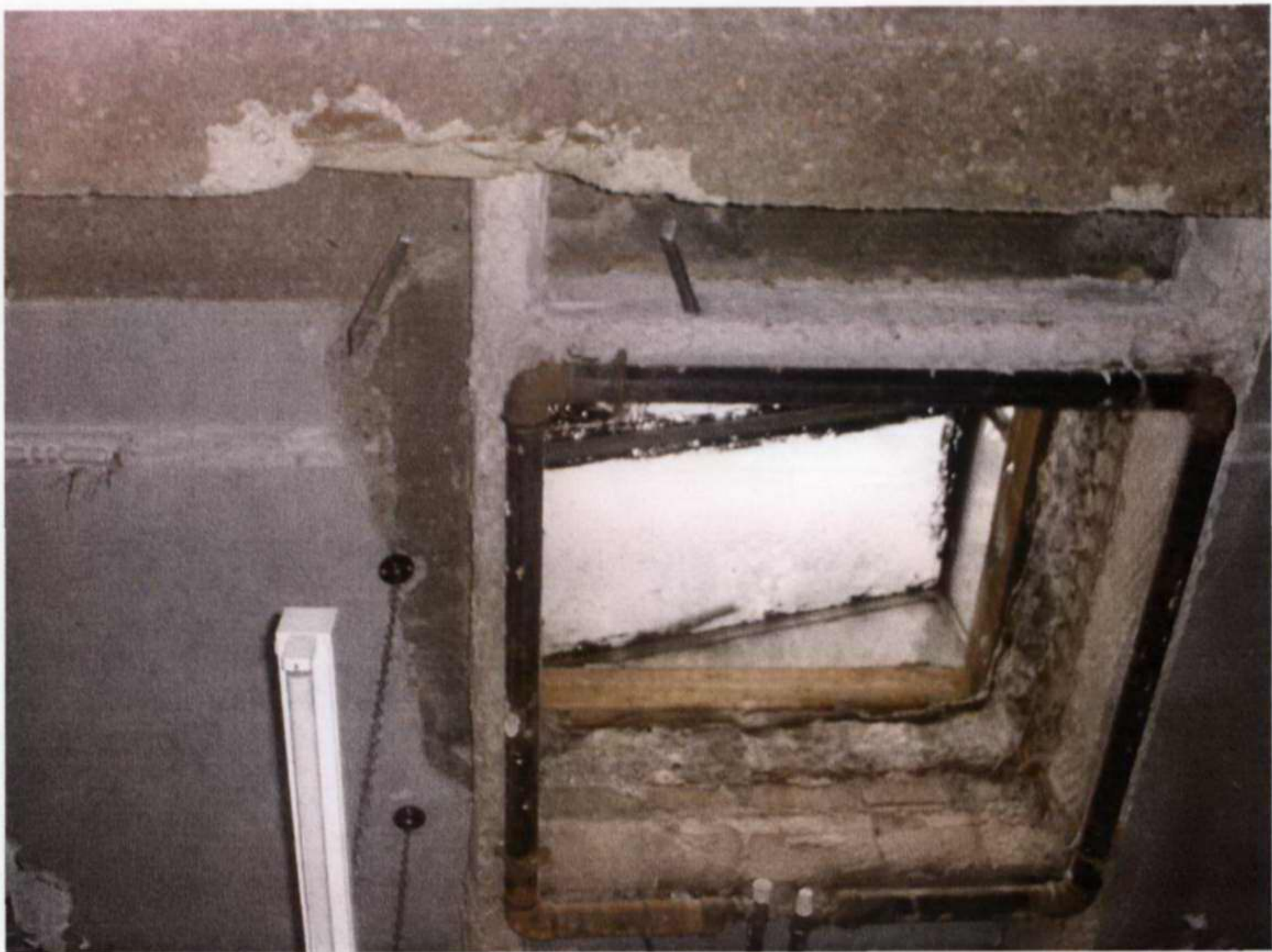
Ref: 006 – View on Roof Light
