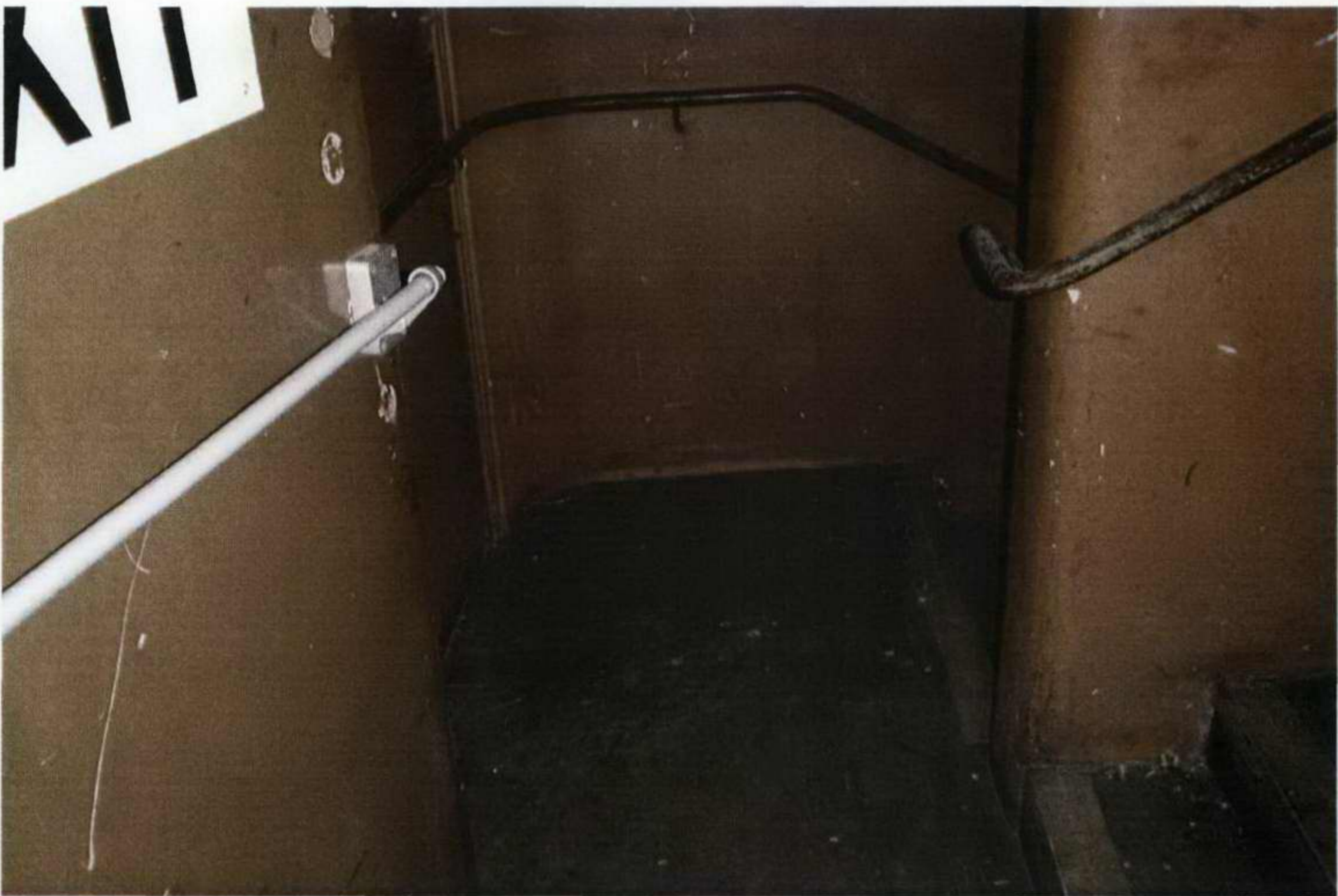
Ref: 008 – View on Emergency Escape Stair
