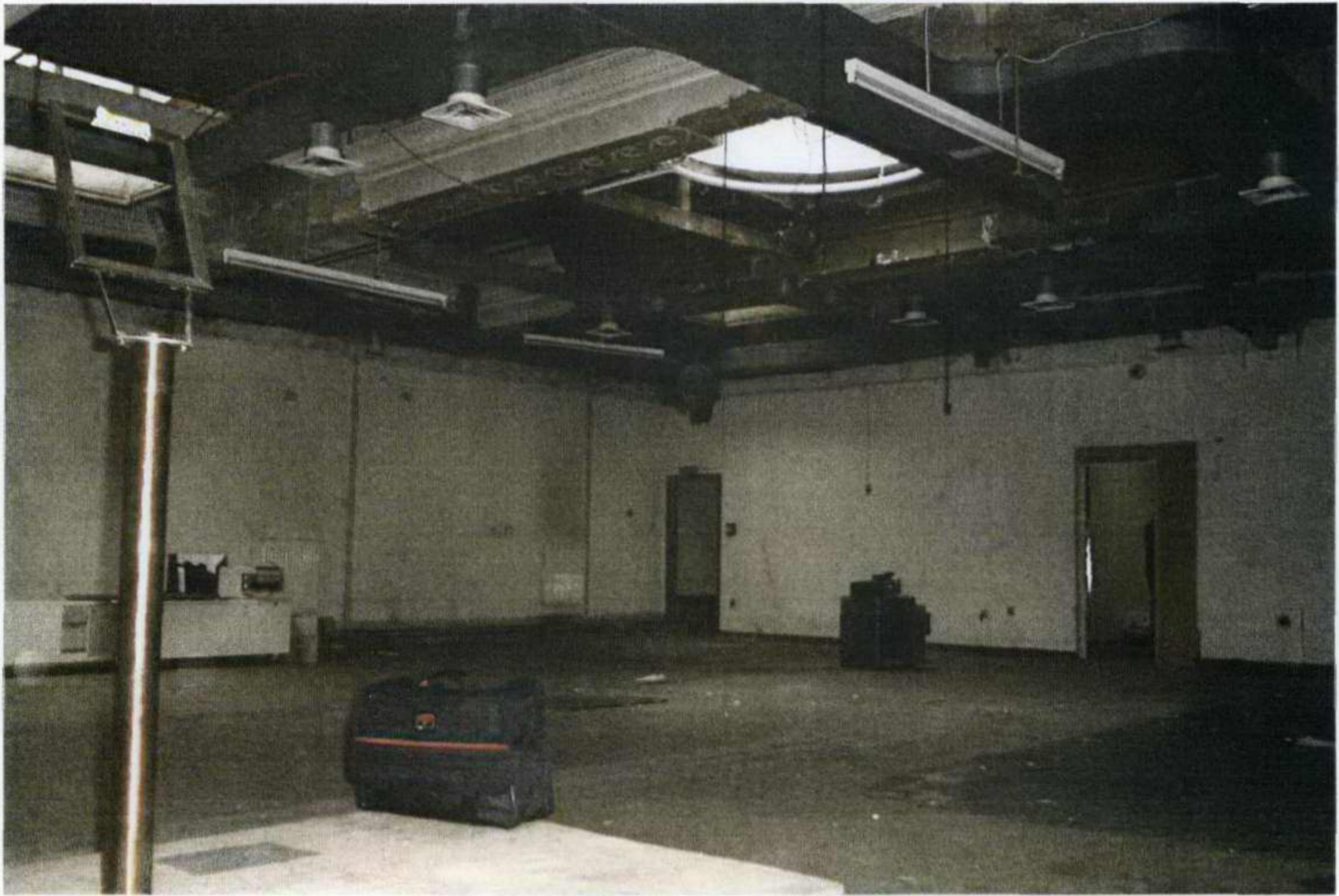
Ref: 007 – General View
