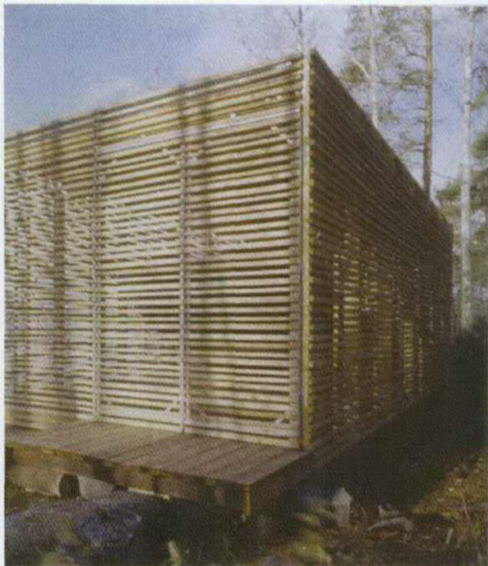
Slatted timber screening
