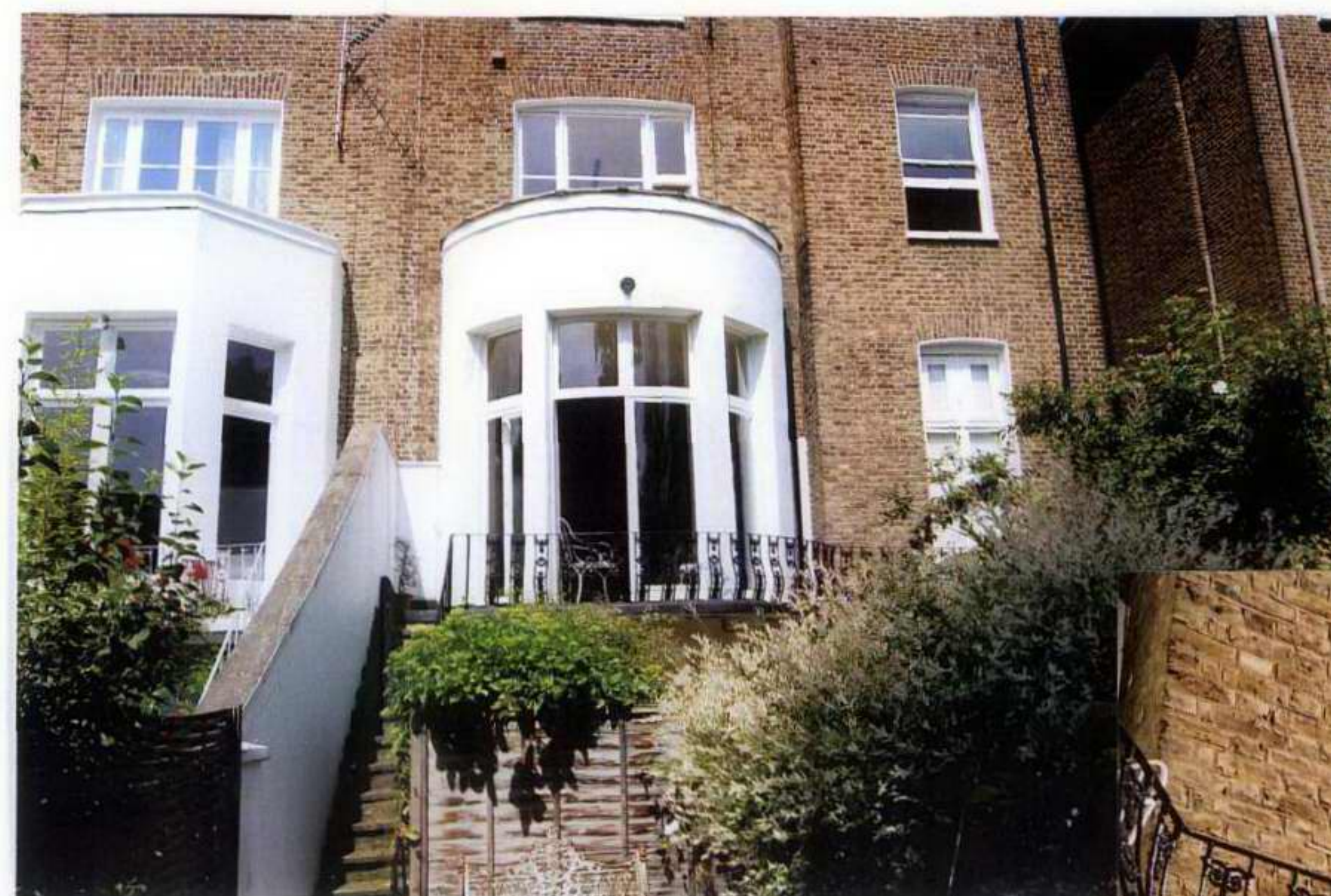
WINDOW TO BEDROOM
