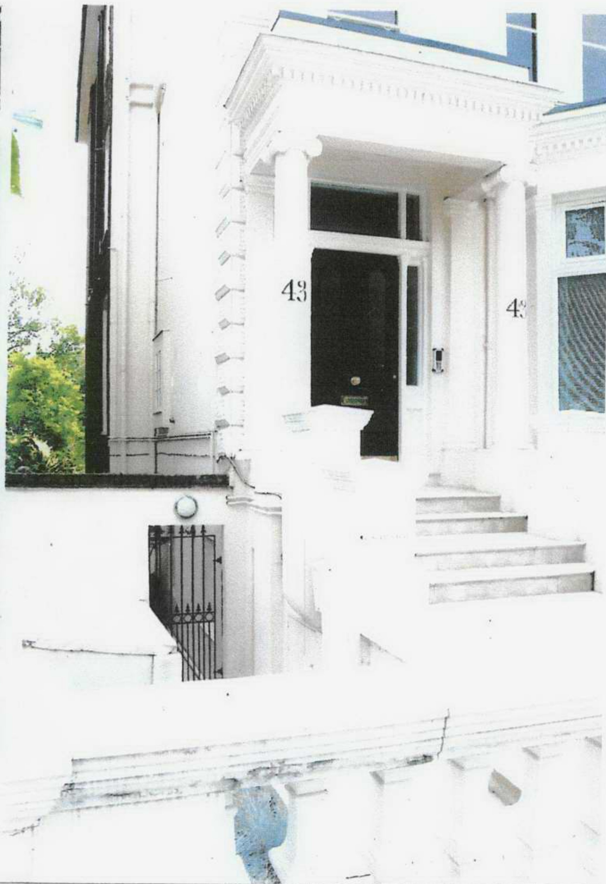
Existing entrance to 43A garden flat through stairs downwards
