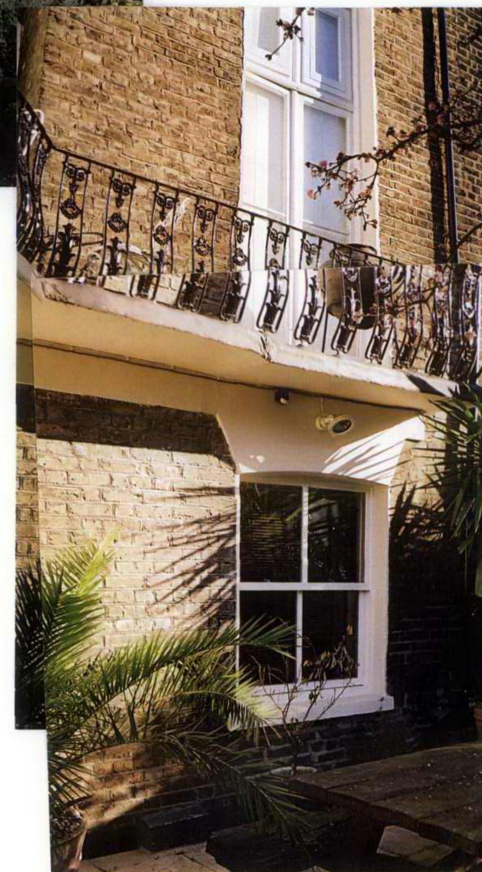
EXISTING WINDOW TO BEDROOM
