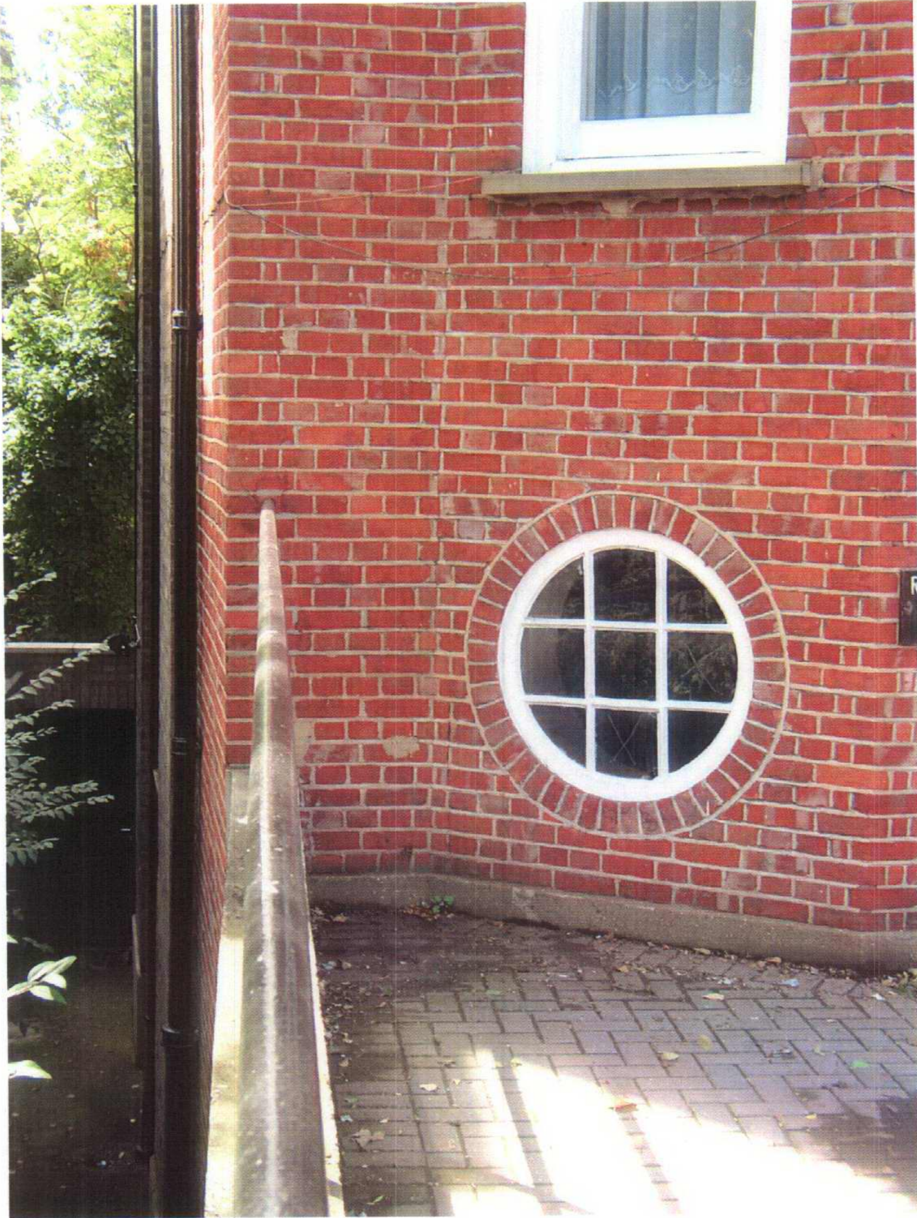
North-east facing wall
