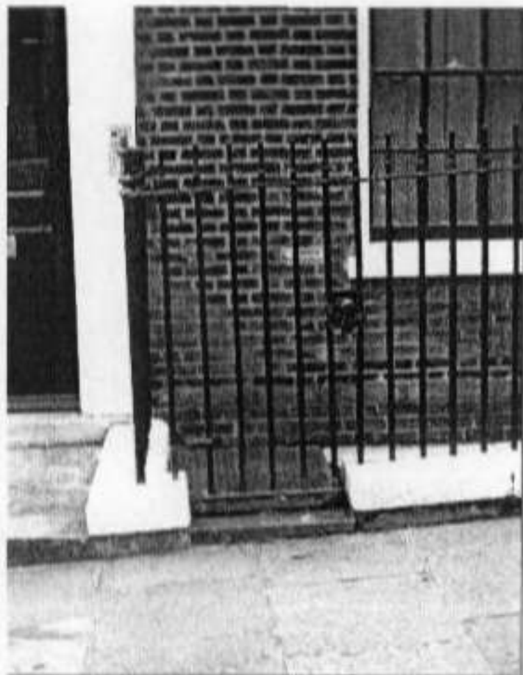
Photo. No. 9.4 : Gate and steps to lightwell of 10 New End
