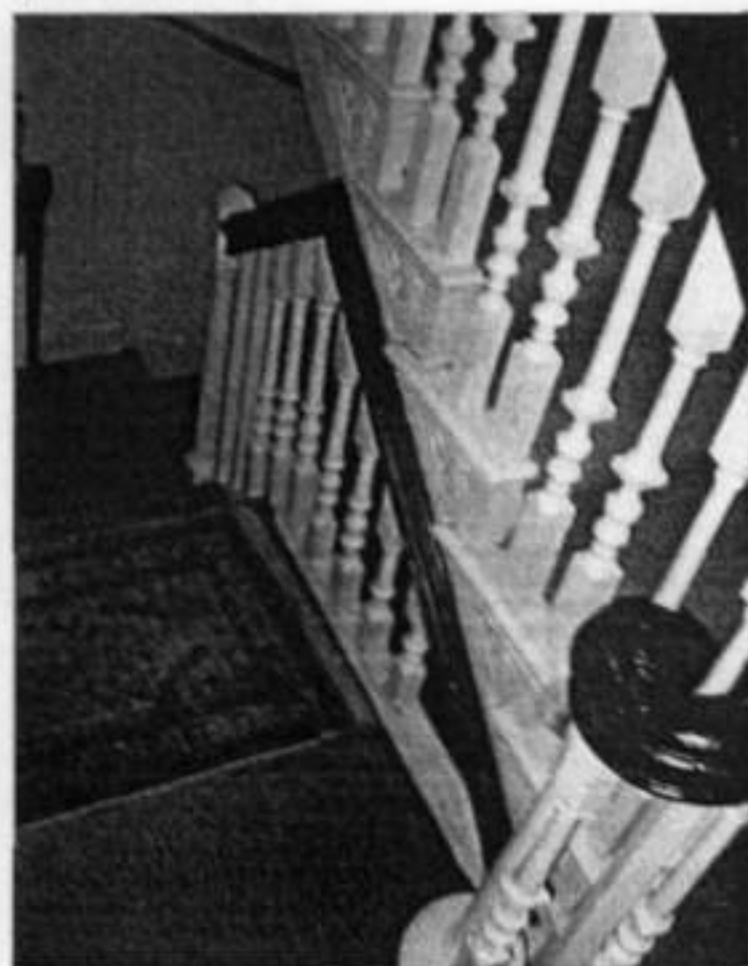
Photo No. 2.3 14 New End - Staircase at ground floor level looking down to lower ground floor
