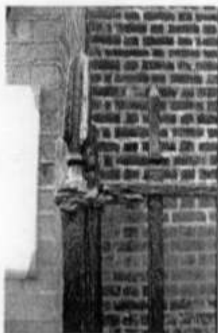
Photo. No. 9.5 : Left hand railing finial, 14 New End.
