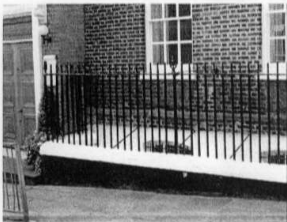
Photo. No. 9.1 : Railings to lightwell of 14 New End
