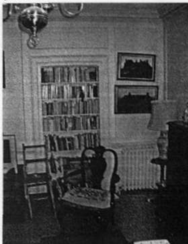
Photo No. 2.4 14 New End - Existing door opening between front and rear rooms
