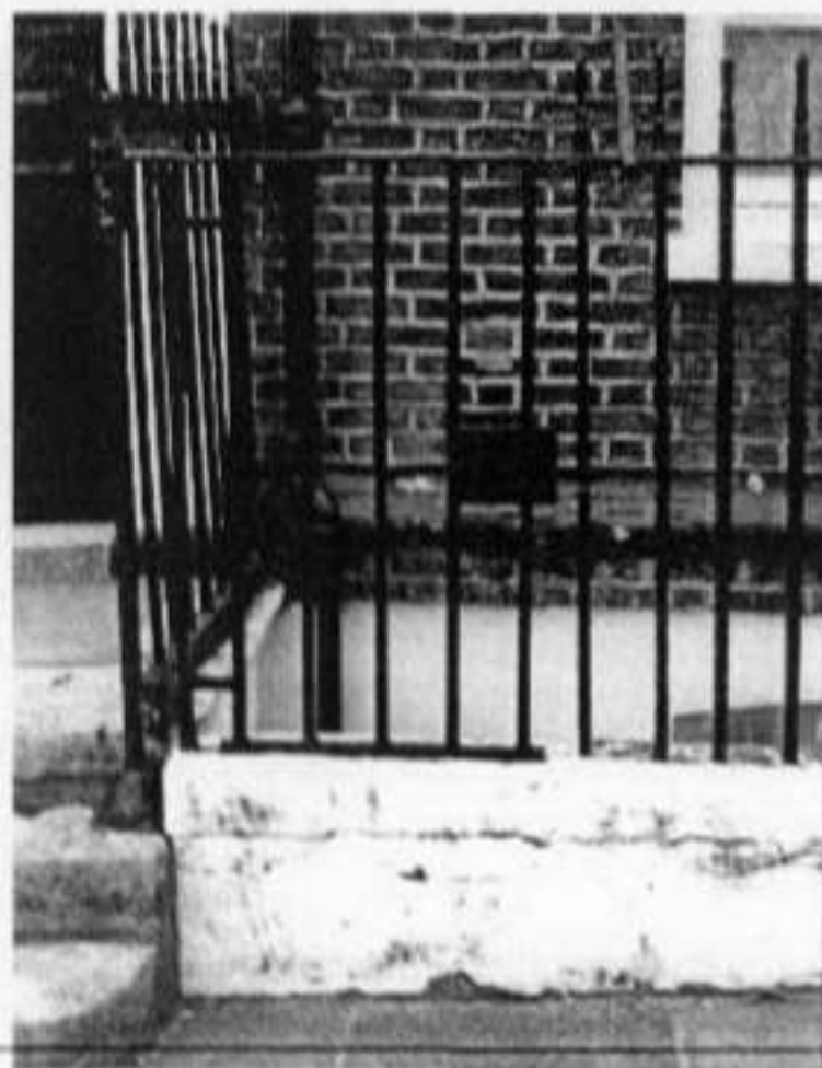
Photo. No. 9.2 : Gate to lightwell of 12 New End
