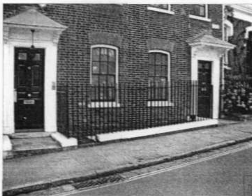
Photo. No. 1.2 Railings to 10 New end including gate and steps to front area.
