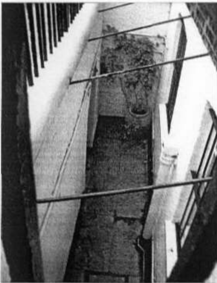
Photo. No. 8.3 : Lightwell
