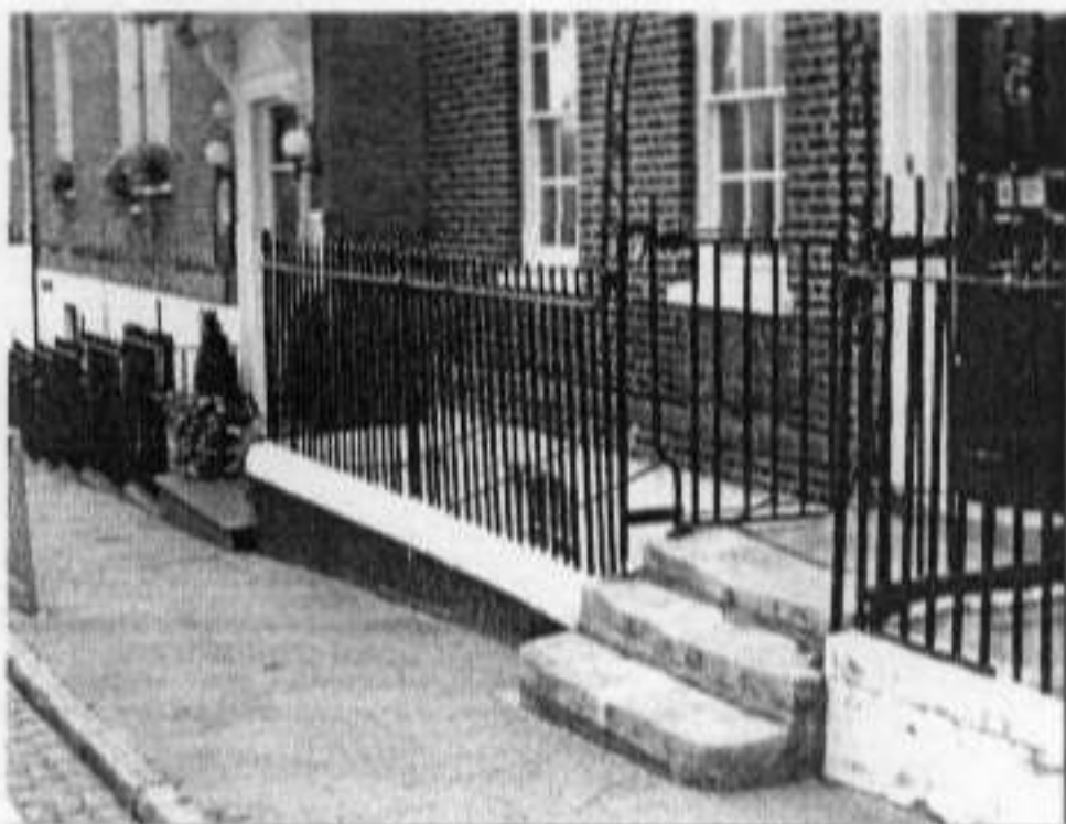
Photo. No. 9.3 : Railings to lightwell of 14 New End
