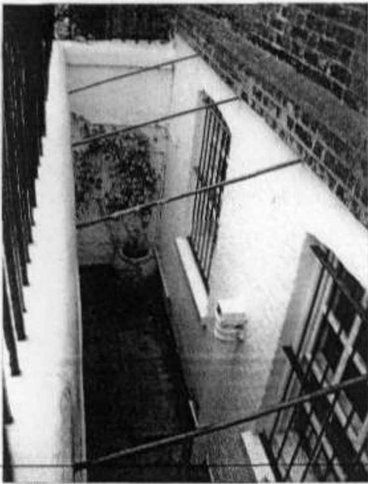
Photo. No. 8.1 : Lightwell
