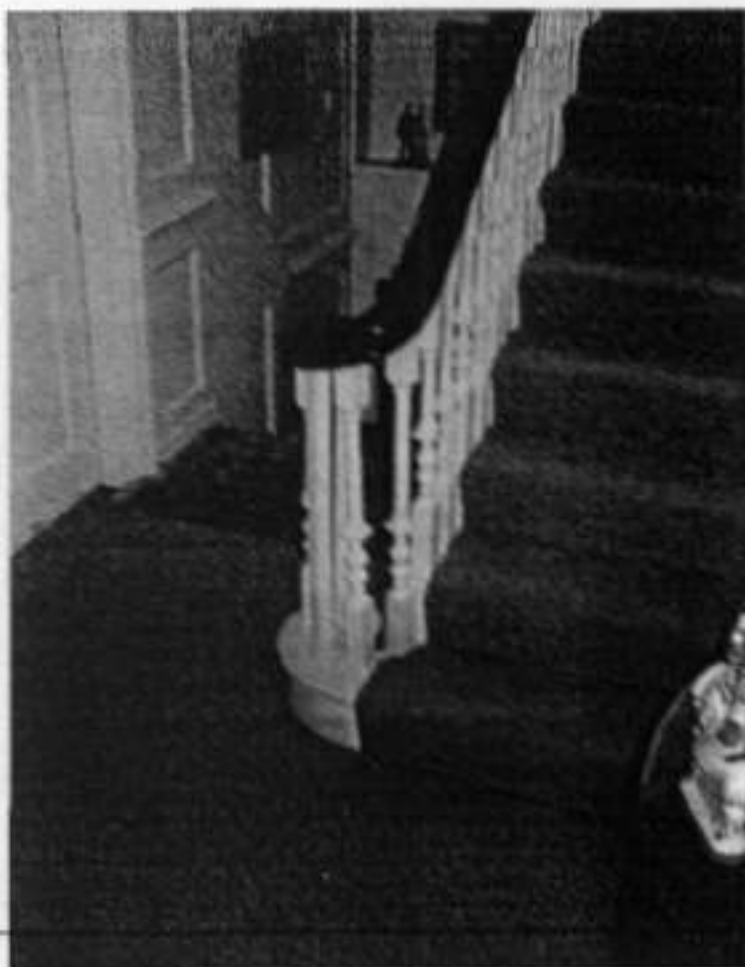
Photo No. 2.2 14 New End - Staircase at ground floor level
