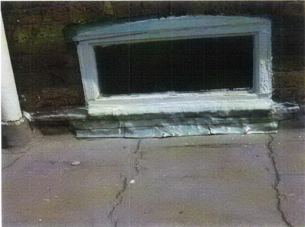
One of two identical windows on the 3 rd floor that will require replacement
