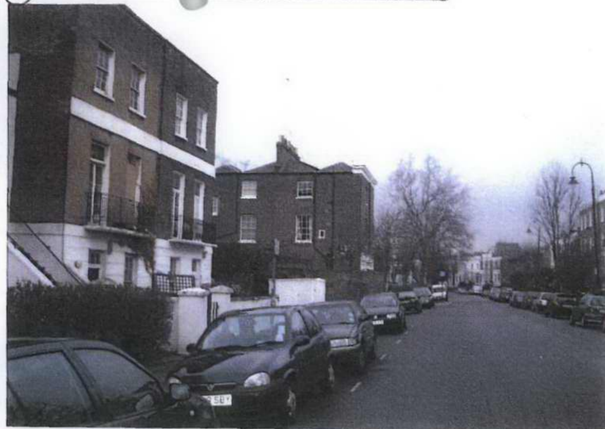
ROCHESTER ROAD LOOKING WEST
