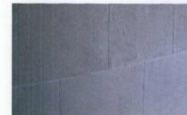
Bromley Reform Synagogue, Memorial Wall. Pitted 'Portofino' polished plaster with course-lines. Customised colour. FRANCO FINISHES
