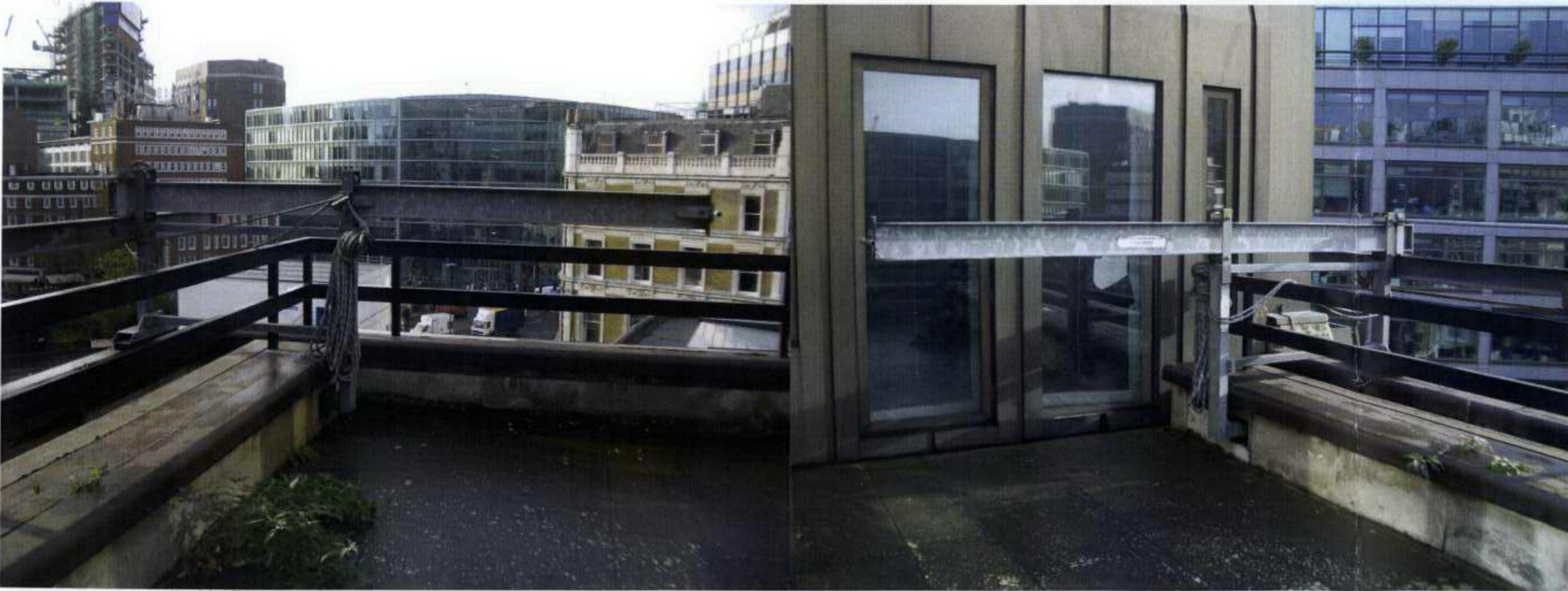
VIEWS OF WINDOW CLEANING APPARATUS ON FRONT (SOUTH) ROOF AREA - TO BE REMOVED
