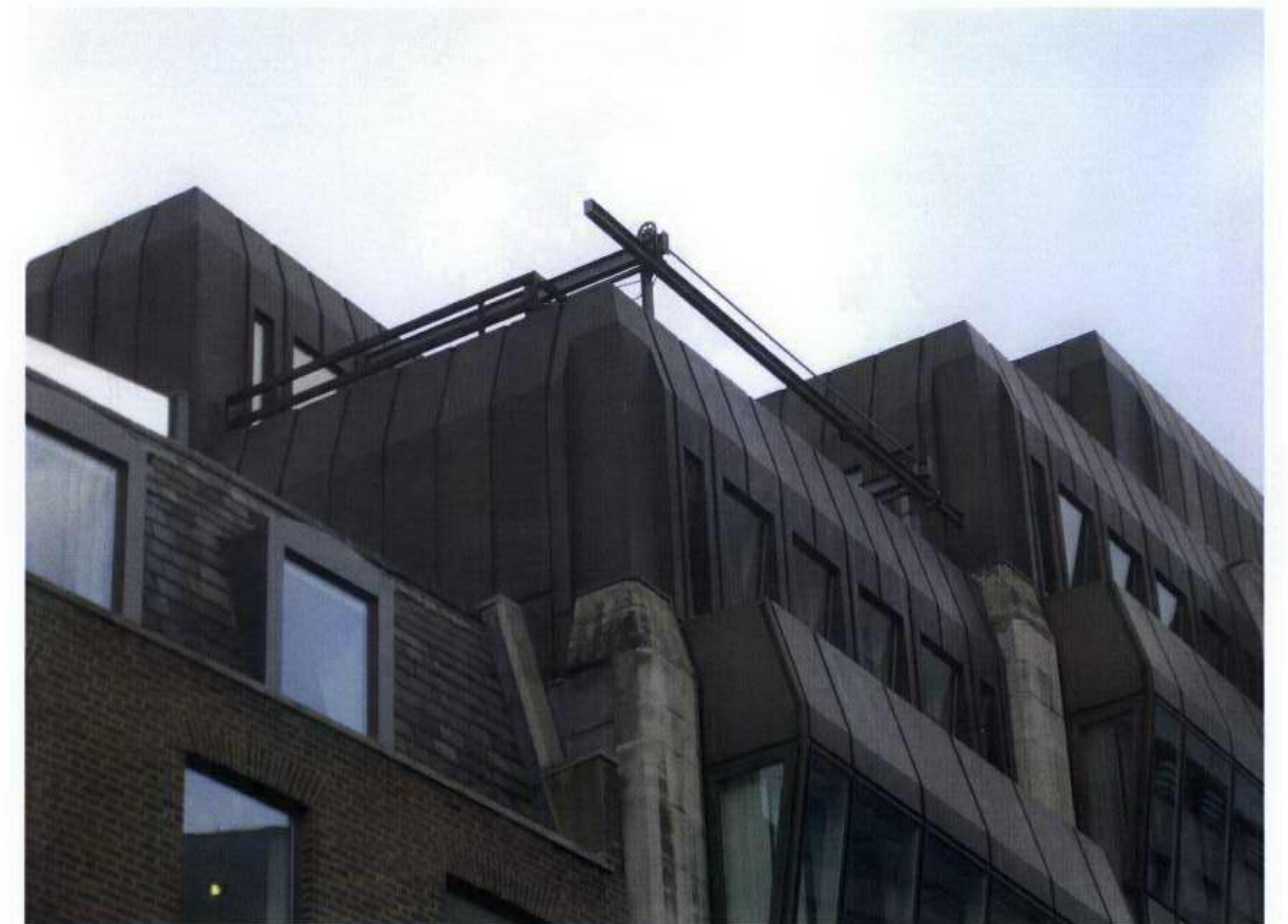
VIEW OF WINDOW CLEANING APPARATUS ON FRONT (SOUTH) ROOF AREA FROM CHARTERHOUSE STREET - TO BE REMOVED
