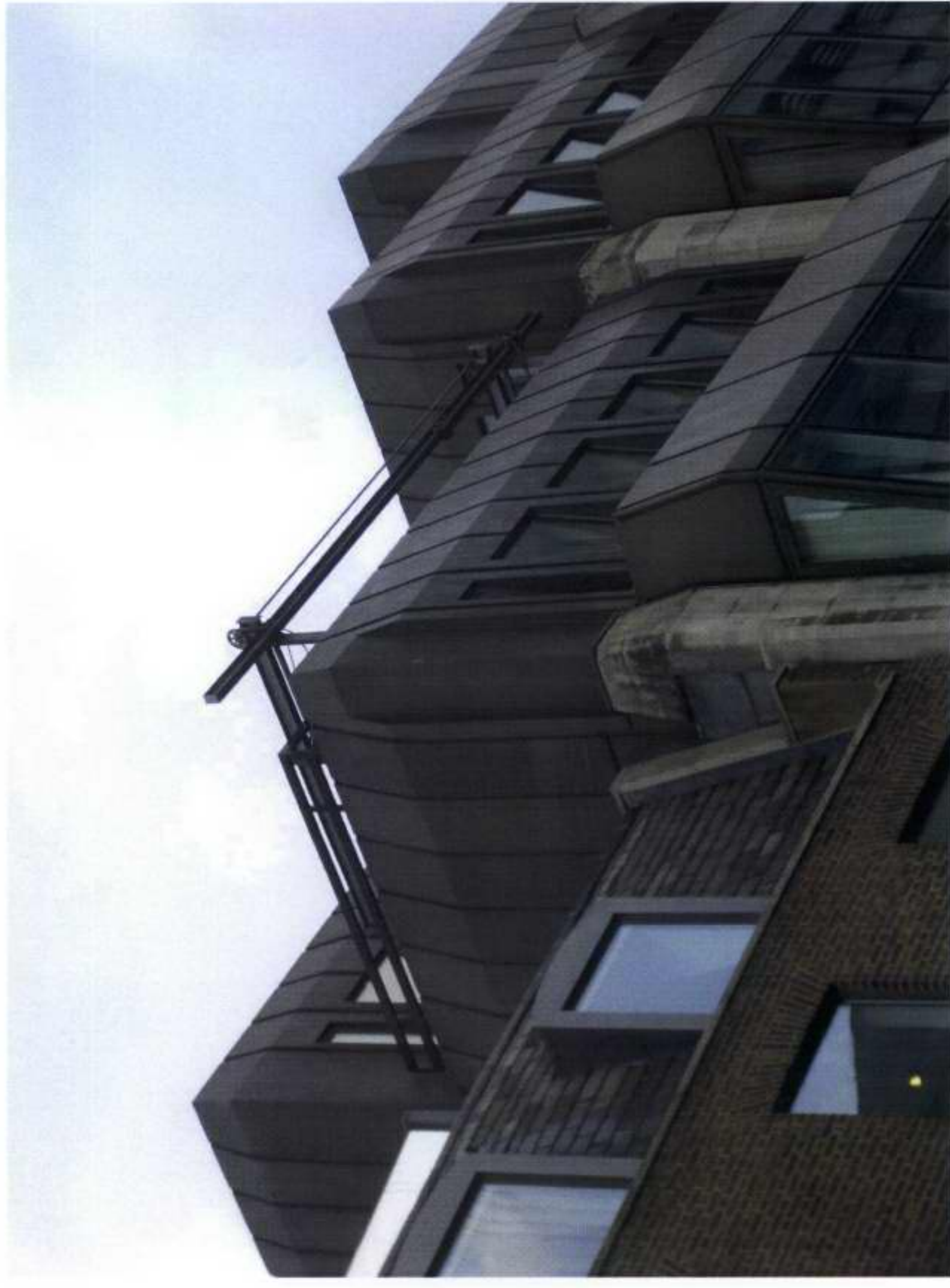
VIEW OF WINDOW CLEANING APPARATUS ON FRONT (SOUTH) ROOF AREA FROM CHARTERHOUSE STREET - TO BE REMOVED
