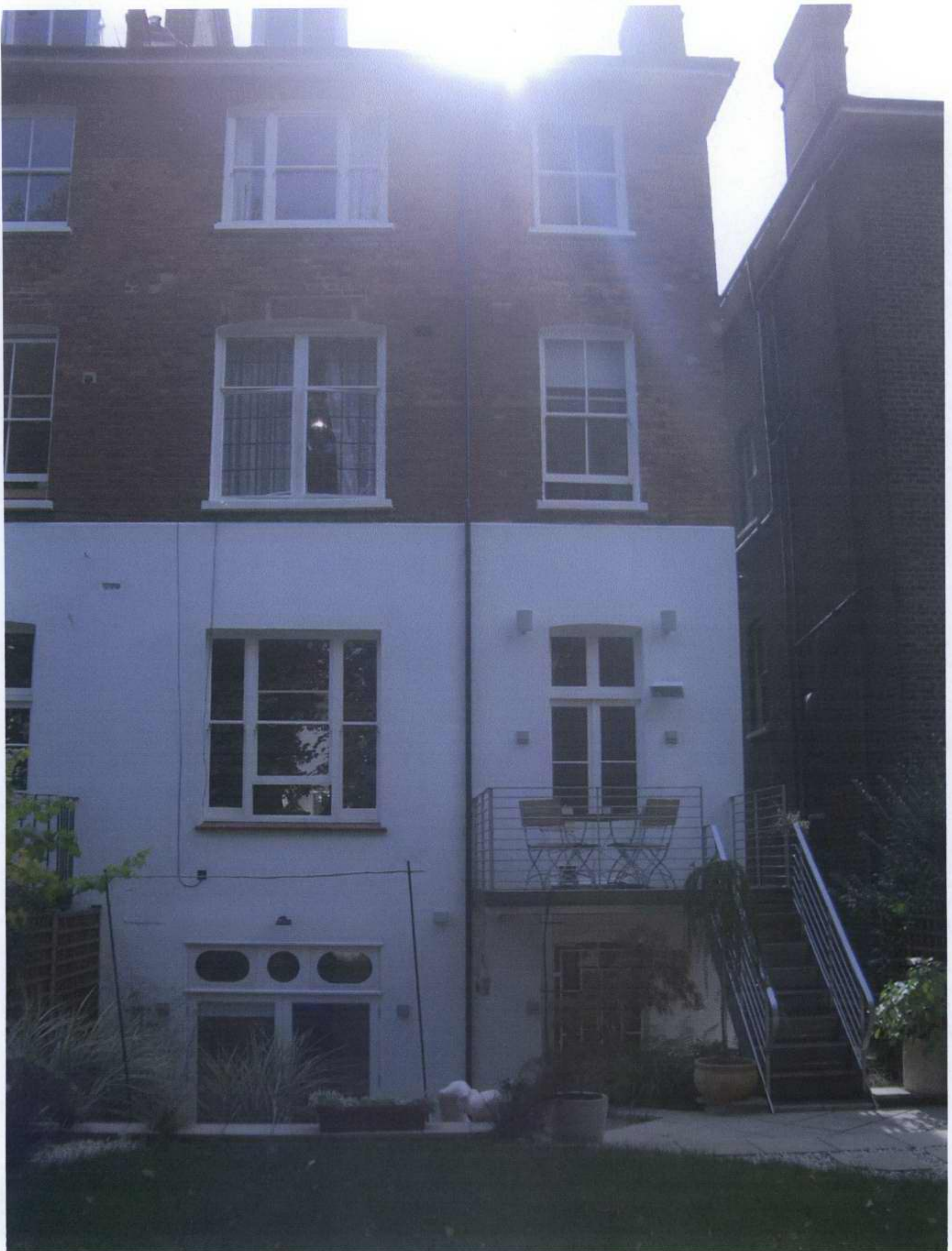
Rear of house showing site of proposed development
