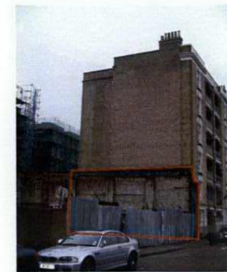
Existing partially-demolished wall to former building on application site to be demolished and replaced with new external wall to proposed building
