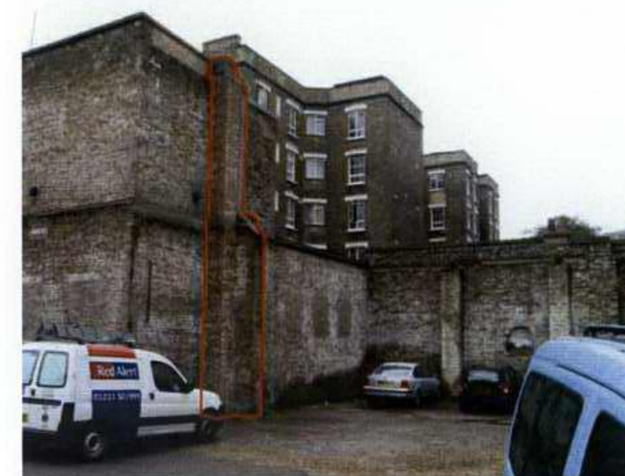
Existing piers to boundary wall at rear of 7-11 Britannia St to be partially demolished to suit new building external wall position
