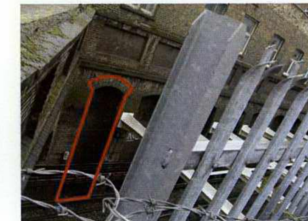
Piers and recesses to railway cutting structure
