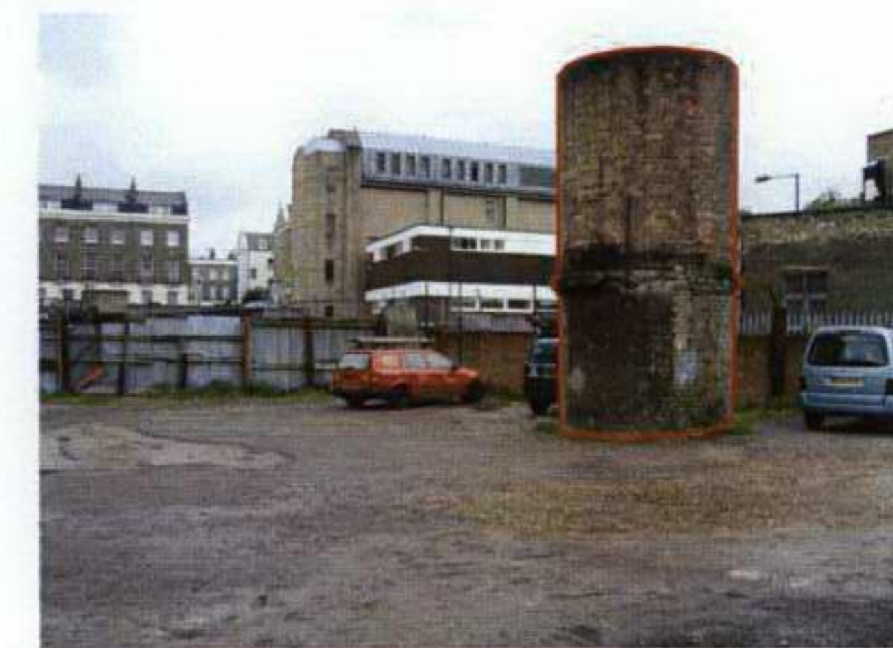
Existing brick tunnel vent to be demolished and capped at ground level to create space for landscaped area
