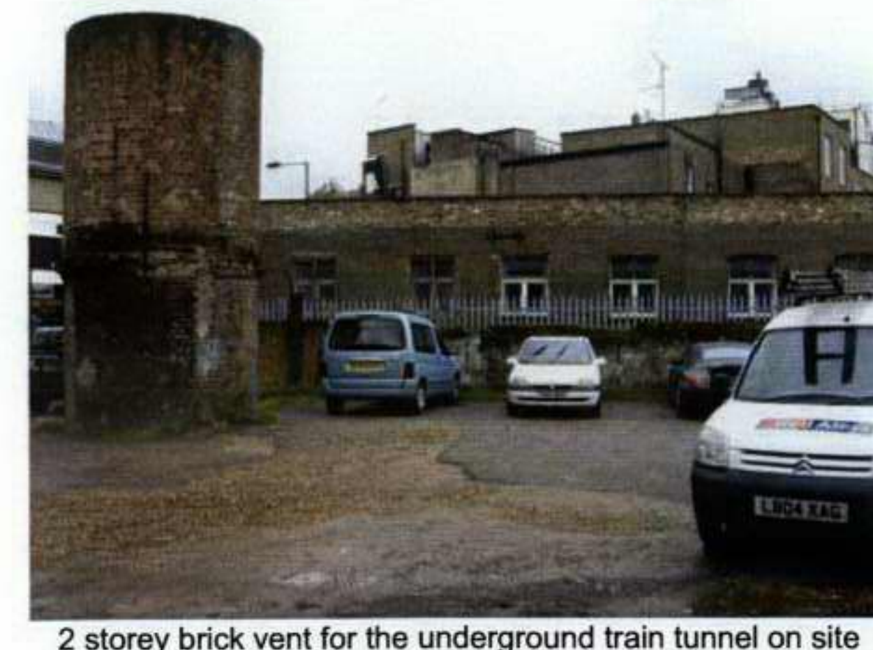
2 storey brick vent for the underground train tunnel on site
