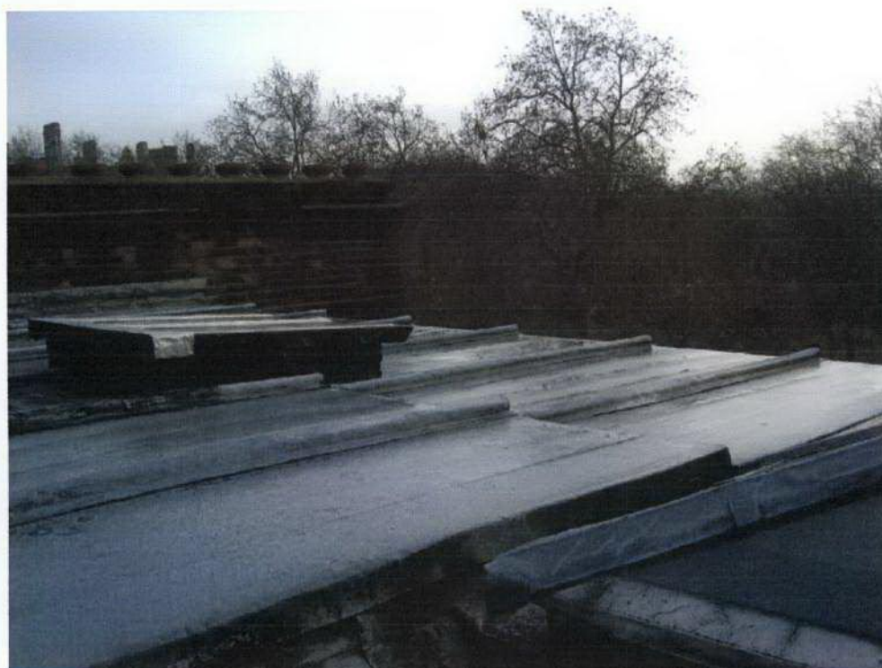
2: Upper rear roof over no.21 without edge protection
