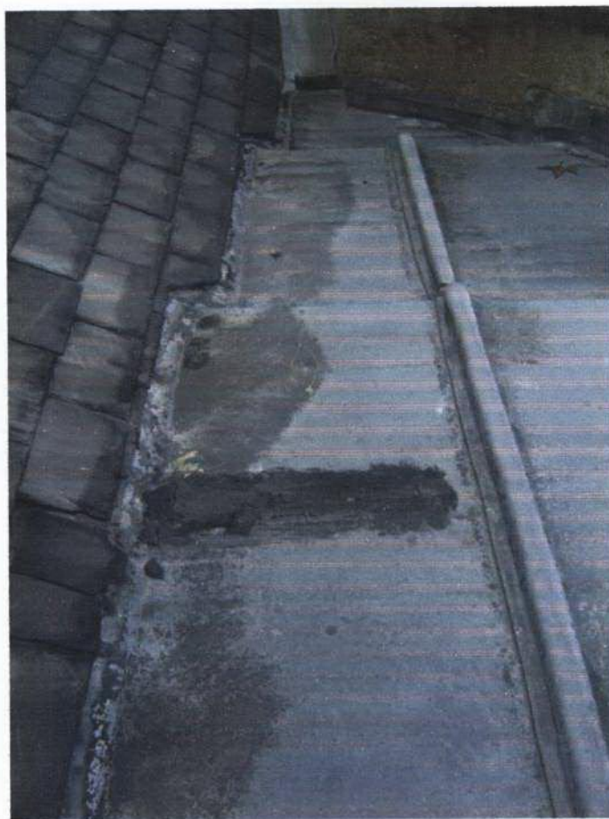
13: Depressed areas and defective leadwork on the lower roof to no.22
