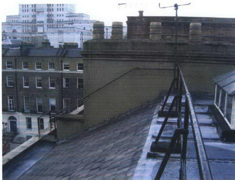
14: Defective render to shared chimney stack with no.23
