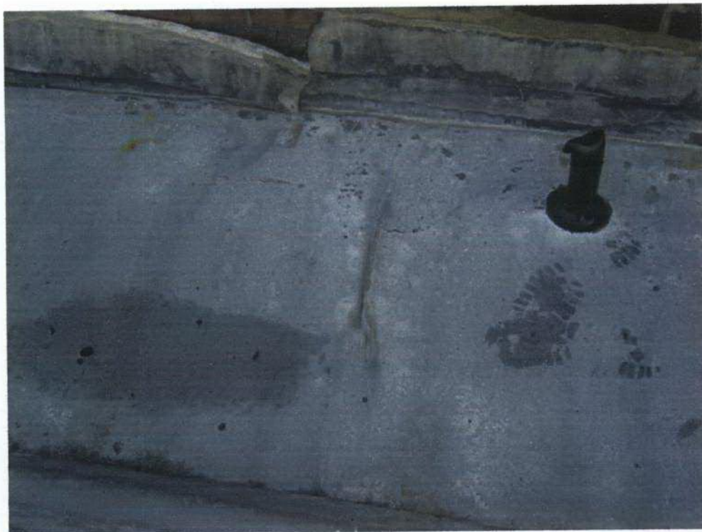
10: Loose flashing and rucked lead sheet over no.22
