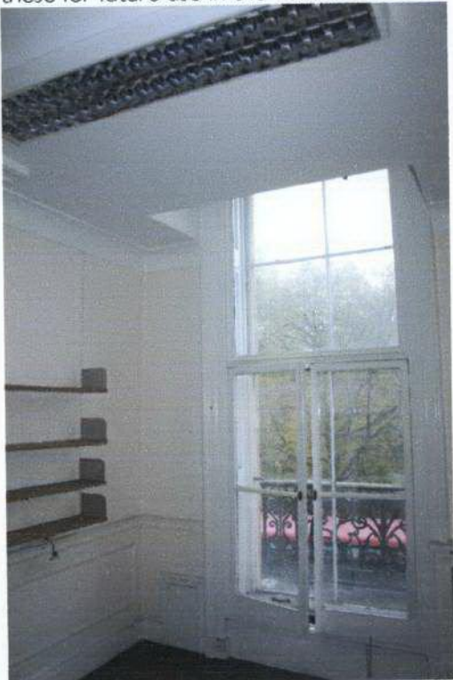
Photo 28 No 22 First floor front rooms typical modern false ceiling to be removed.
