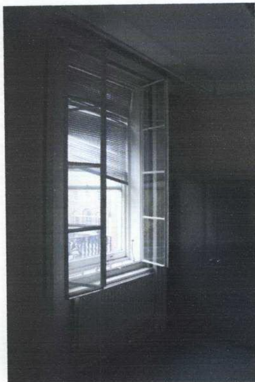
Photo 40 No 21 2 nd floor front window Note Inner glazing to be removed.
