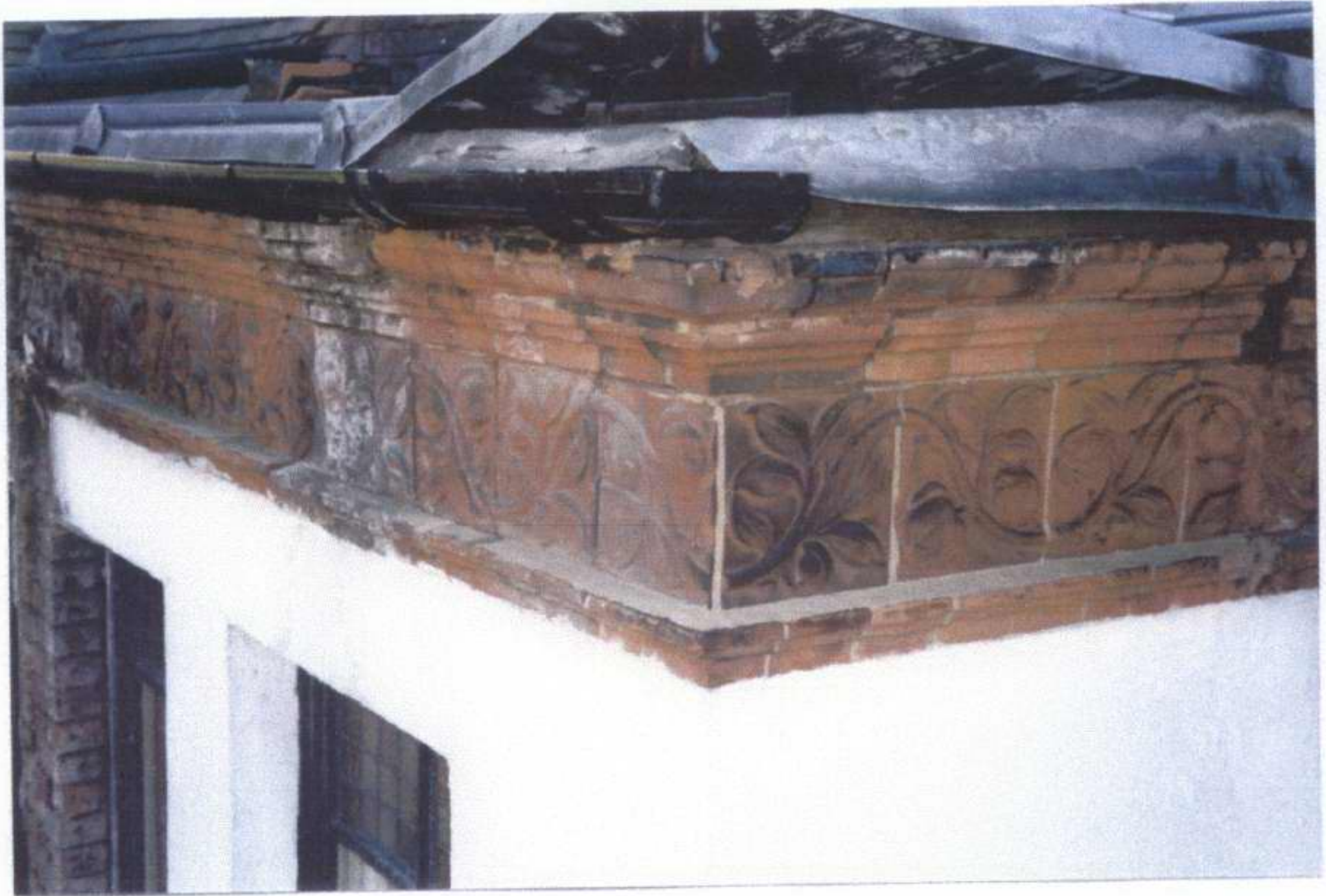
Photos of terracotta band courses with replicas to be used on new building
