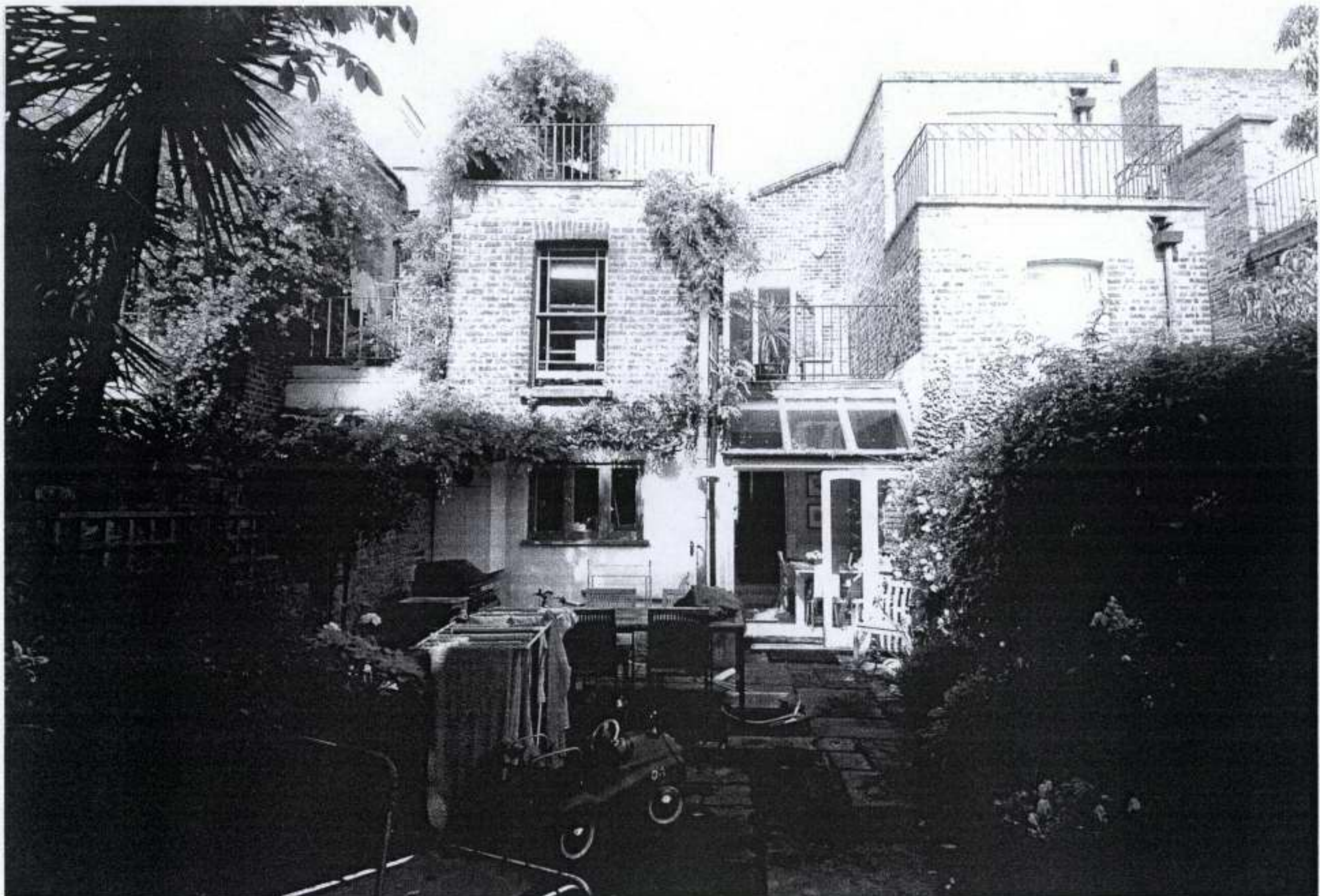
Rear elevation (South East) of 18 Harmood Street NW1
