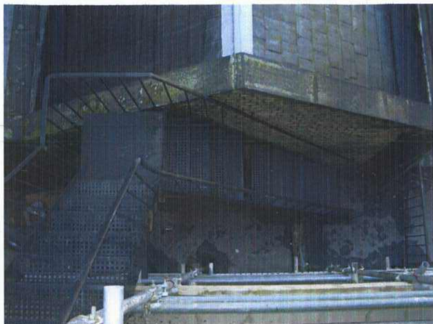
VIEW WEST DOWNWARD 1 SK 21
