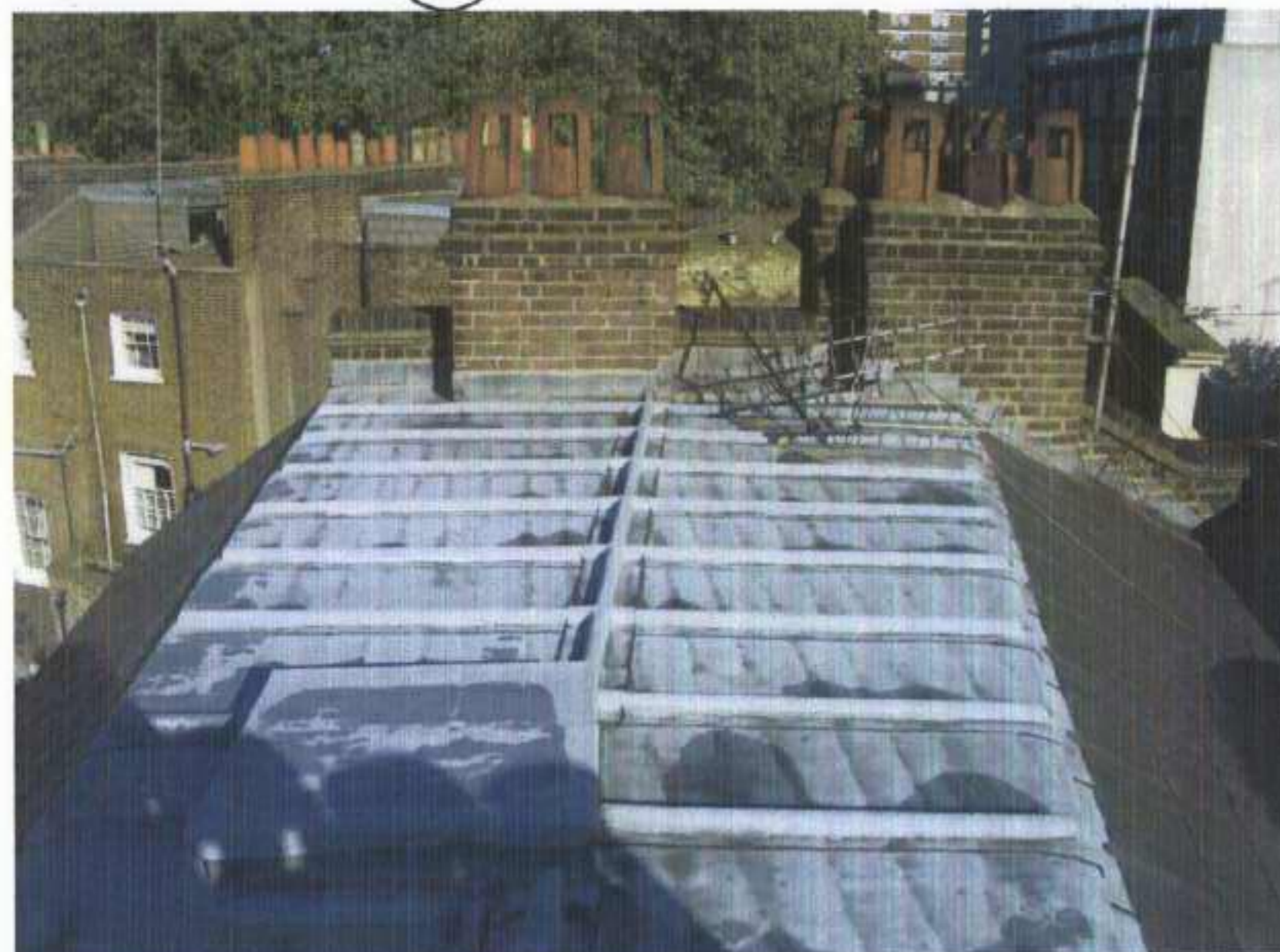
VIEW NORTH 3 SK 21
