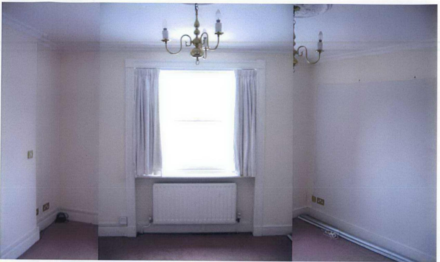
Existing 10mm carpet, 4mm hardboard and chipboard flooring to be removed.
