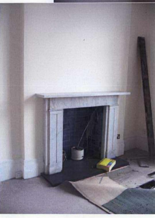
Existing 10mm carpet, 4mm hardboard and 22mm floor boards to be removed.
