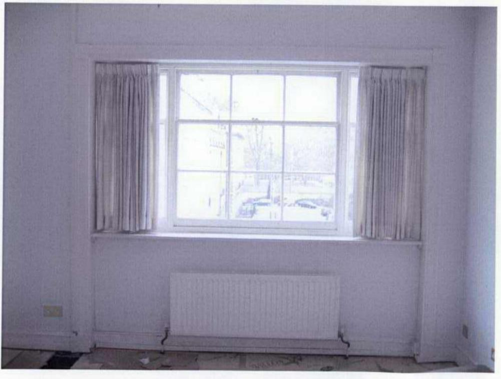
Existing 10mm carpet, 4mm hardboard and 22mm floor boards to be removed.
