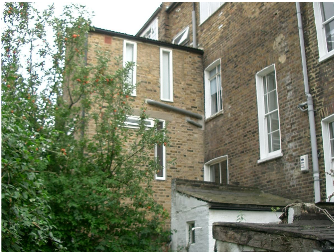
View at Existing 3.5 Story Rear Extensions at 179 Leighton Road
