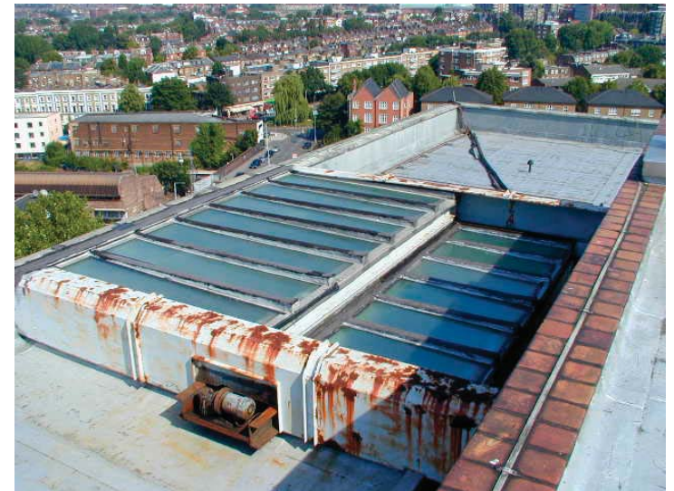
Site Photos - Roof
