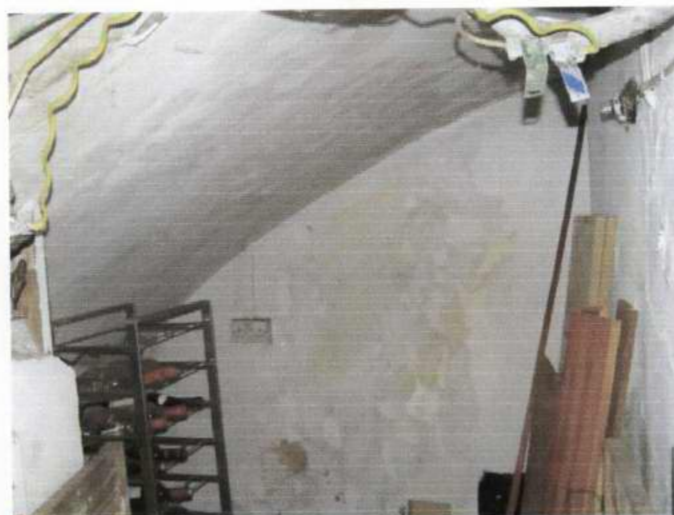
10. View of existing vault space.
