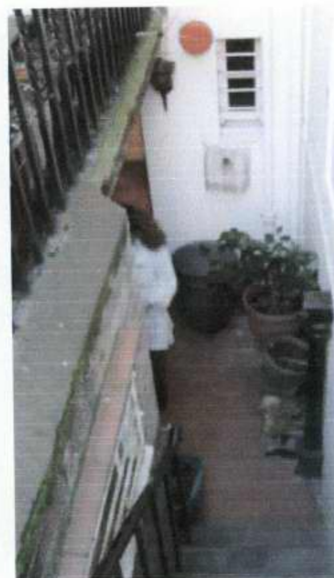
02. Existing basement patio from street.
