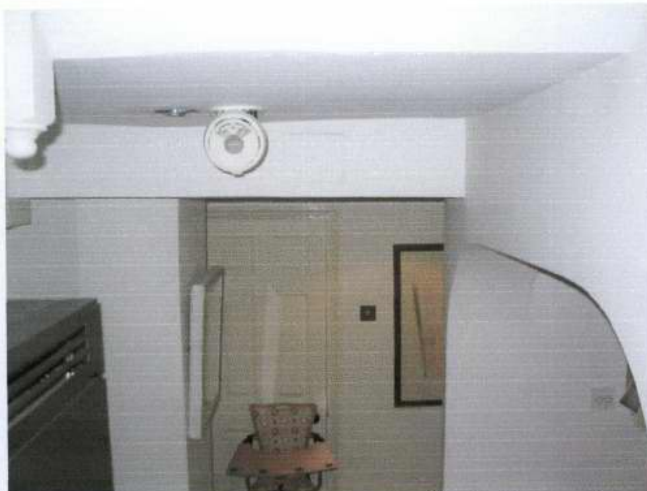
13. Internal view showing existing boxings at ceiling level –no cornices.
