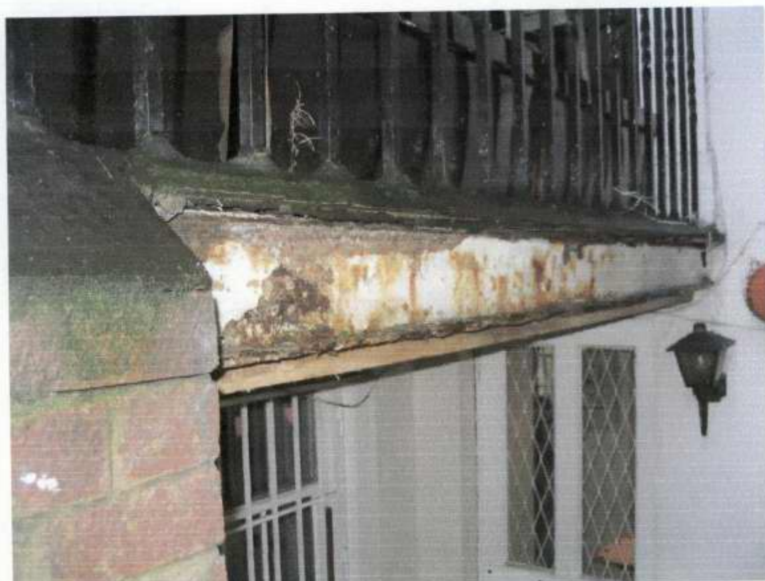
01. Existing concrete slab (bridge) in hazardous conditions
