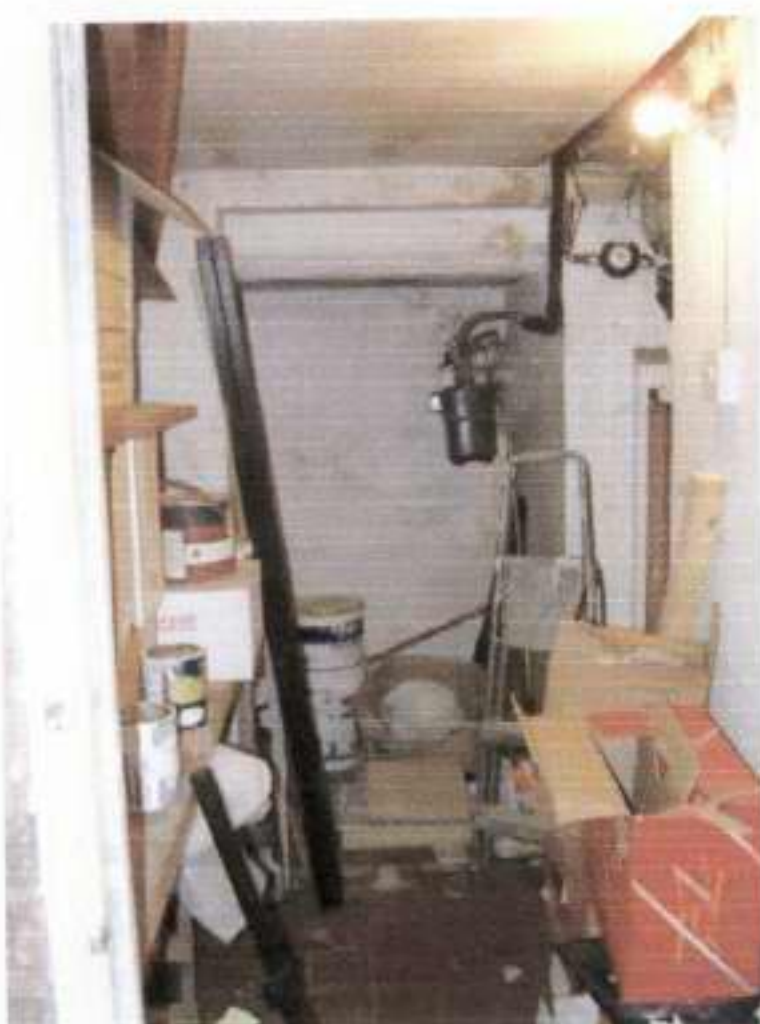
09. View of existing vaults under entrance bridge
