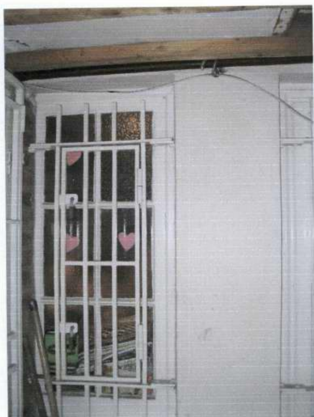
03. Existing Basement (Kitchen) window 1
