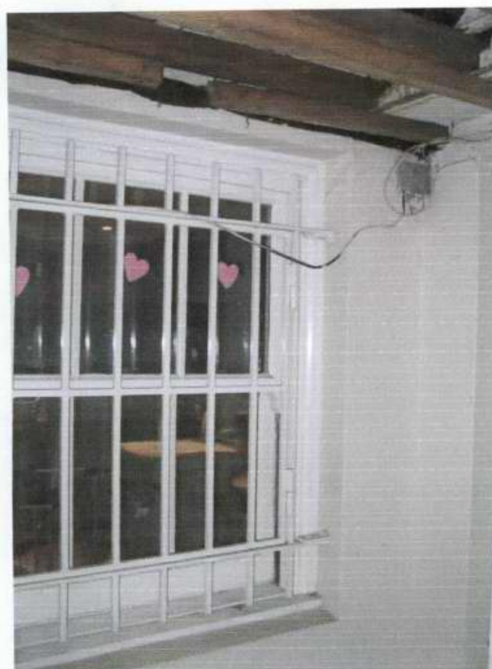
04. Existing Basement (Kitchen) window 2
