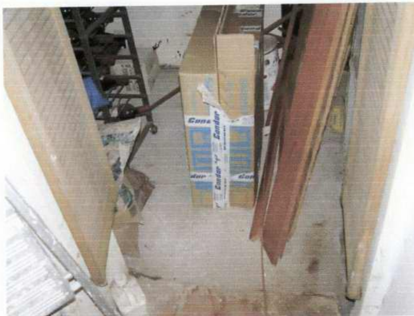
07. View of existing vaults flooring.
