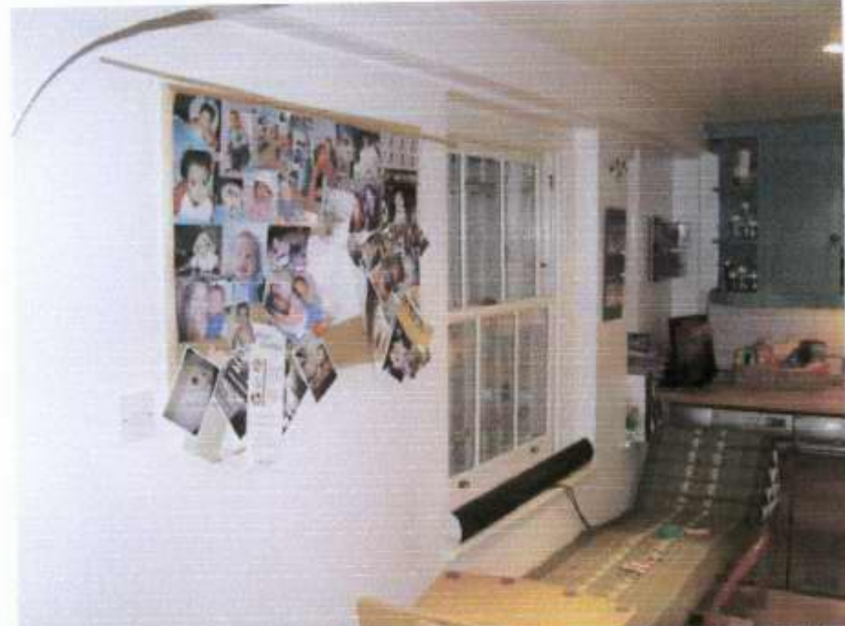
12. Kitchen elevation view showing existing windows. Note existing boxing for water pipework (no cornices).
