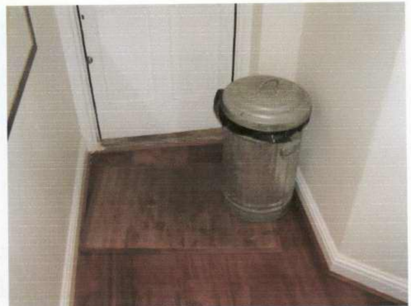
14. Internal view showing non-original flooring and skirting.
