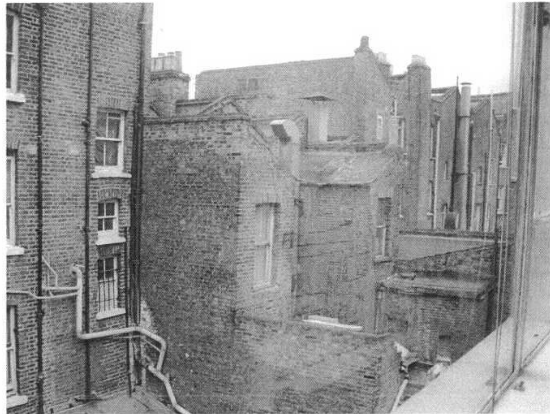
REAR OF BUILDINGS 19-31 CAMDEN HIGH ST
