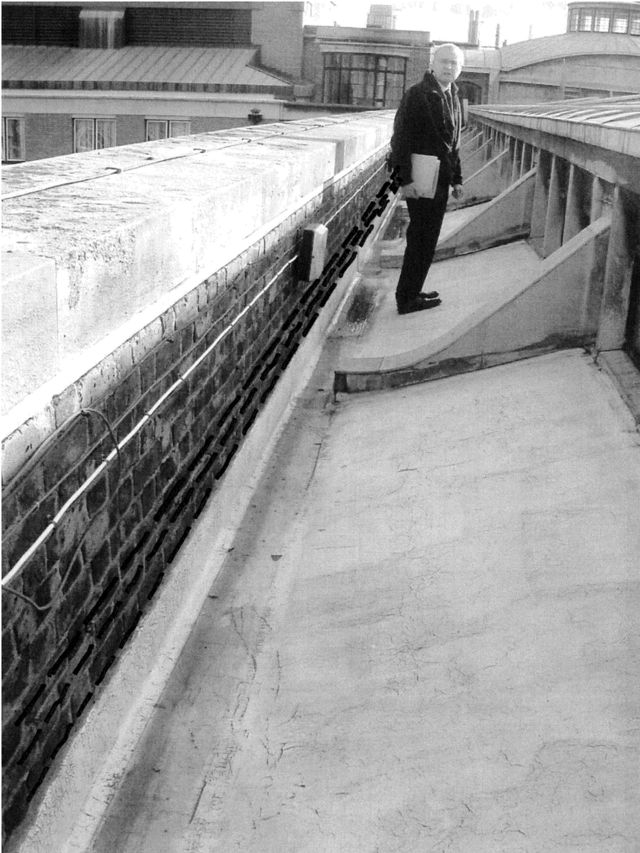
Route for VRF pipework along inner face of parapet - see M&E drawings
