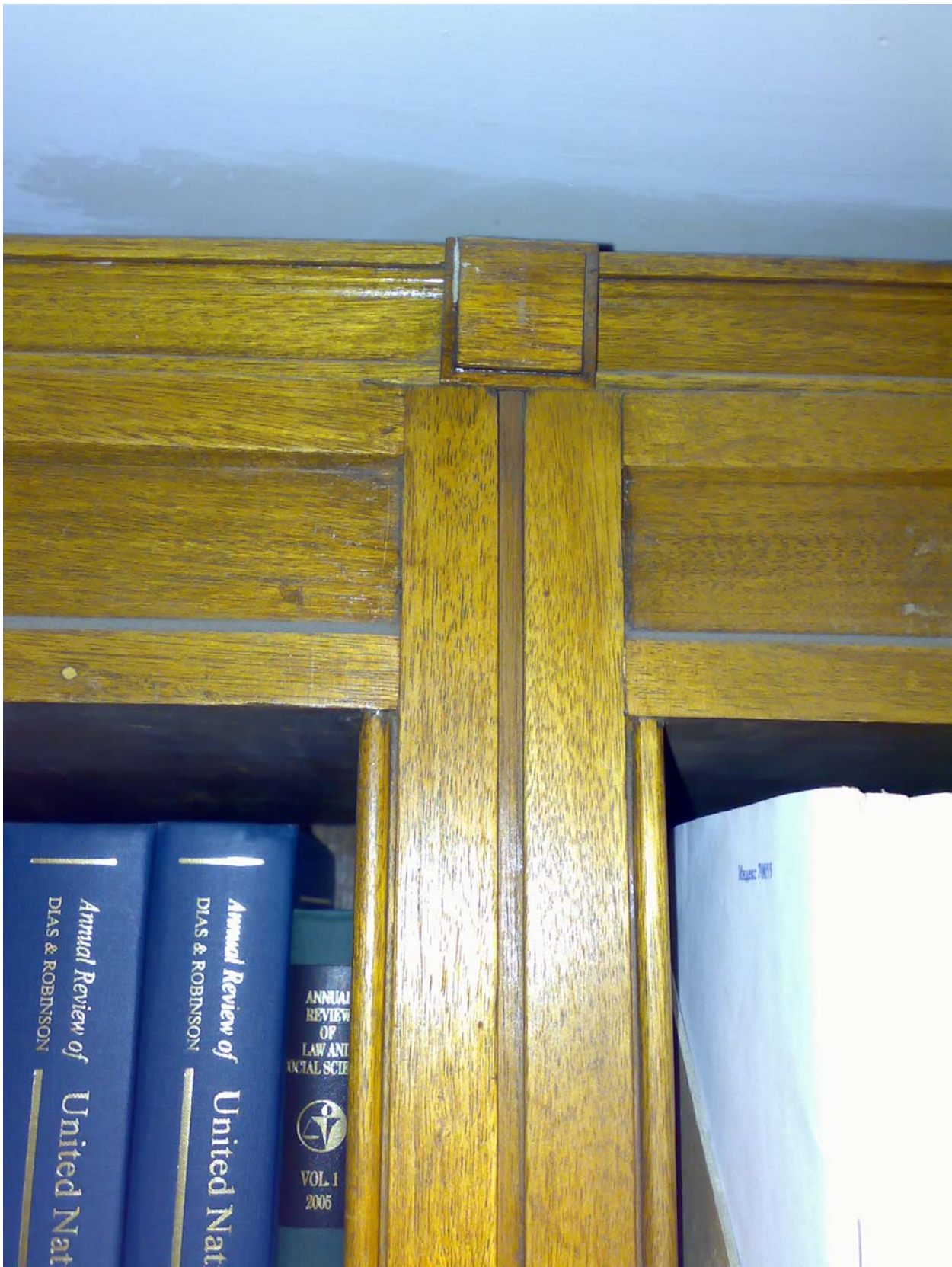
Original connecting dowel between consecutive pelmet
