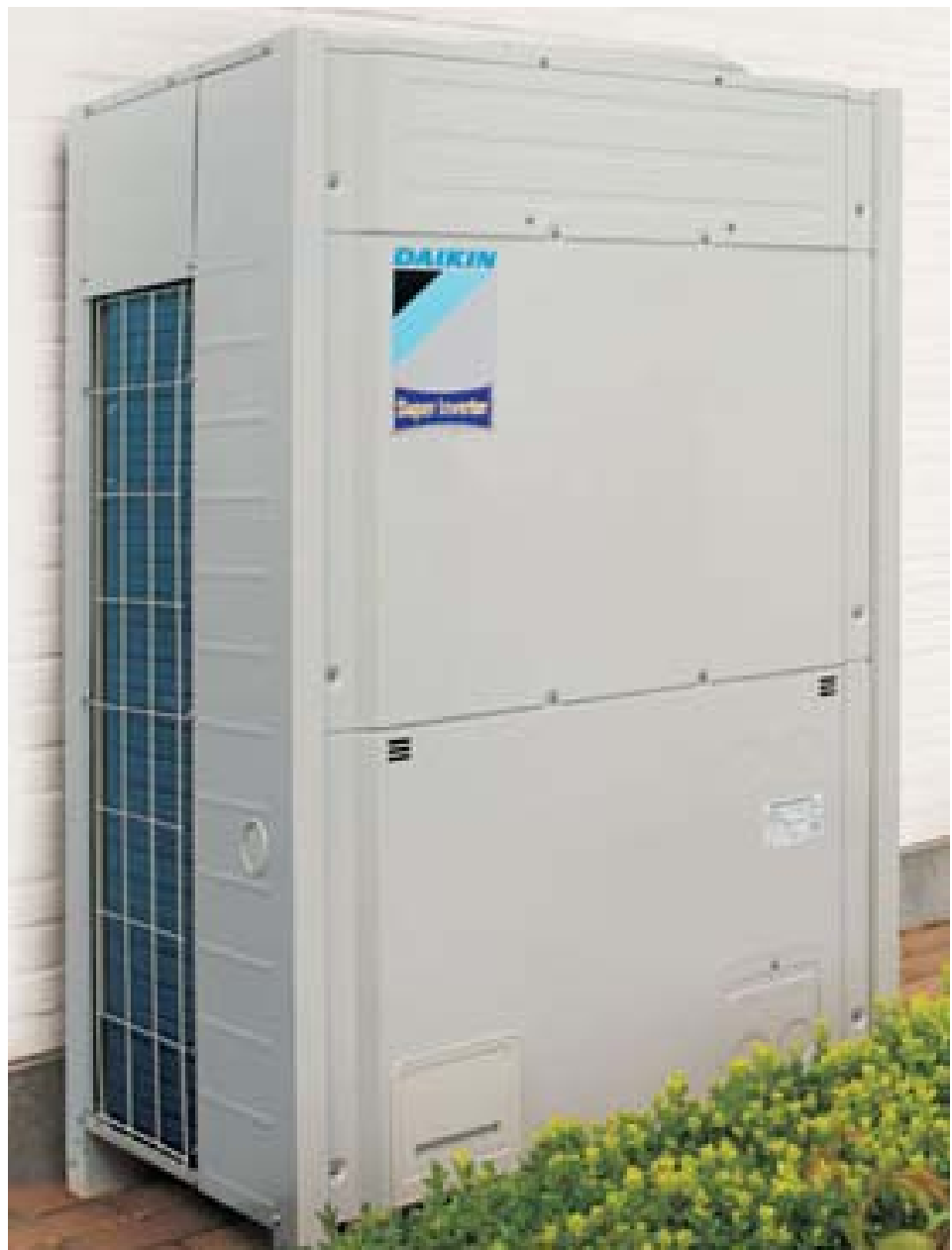
DAIKIN HEAT RECOVERY CONDENSING UNIT (B)
