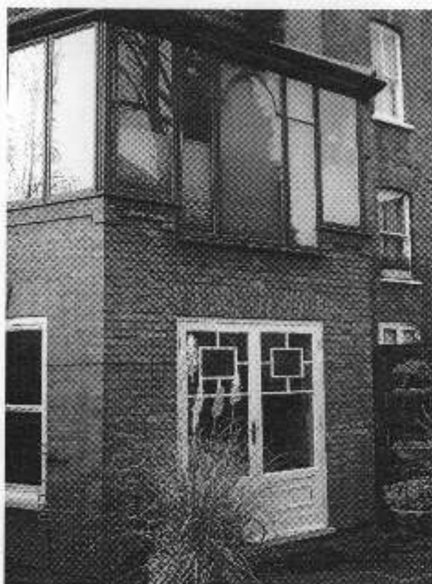
Existing East Elevation Windows / Doors
