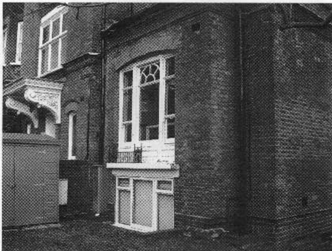
Existing West Elevation lower ground window & lightwell
