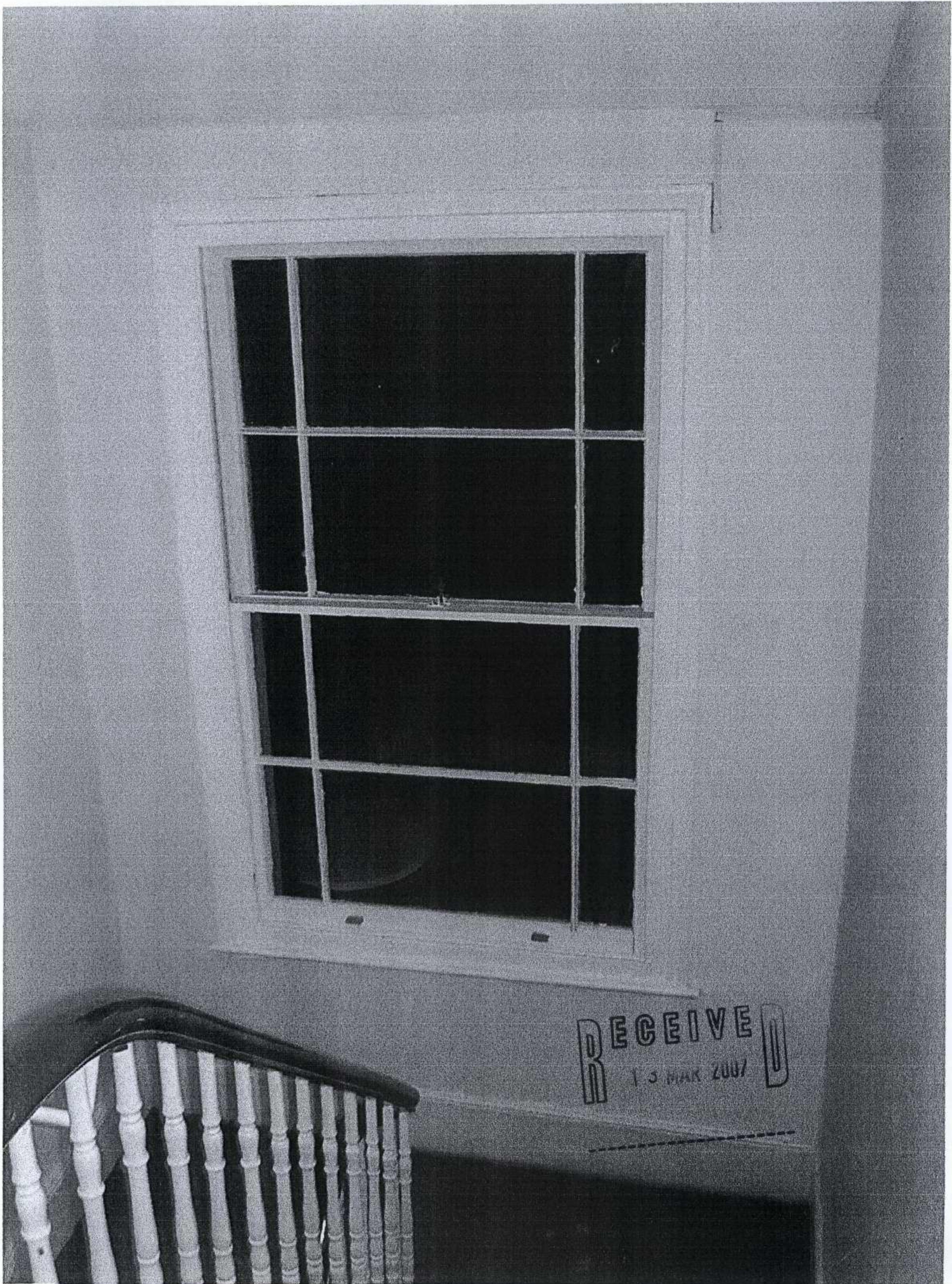
INTERIOR VIEW OF EXISTING WINDOW
