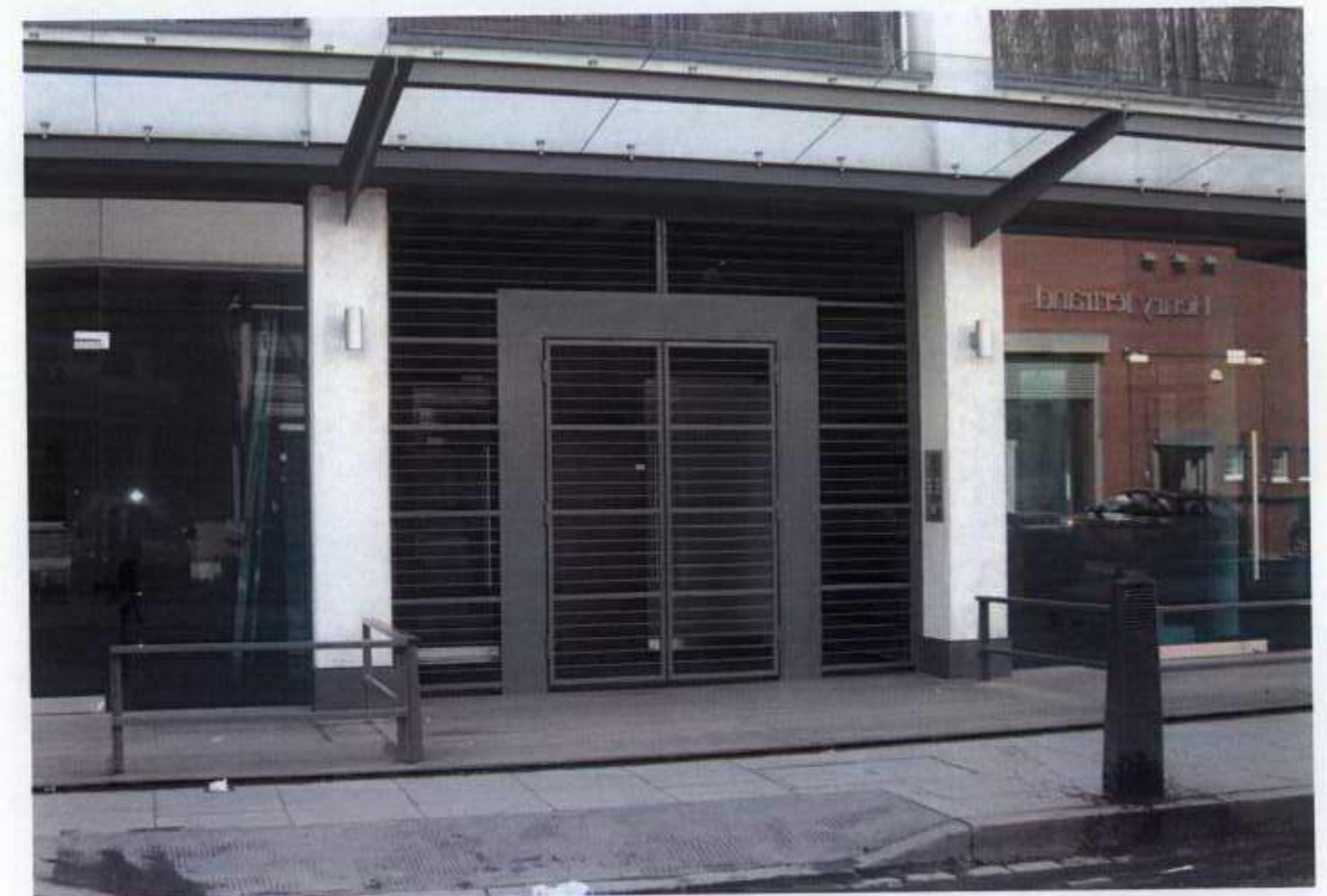
Fig. 5 Photograph showing 40mm step up onto the timber deck at the main entrance to 55 Holmes Road.
