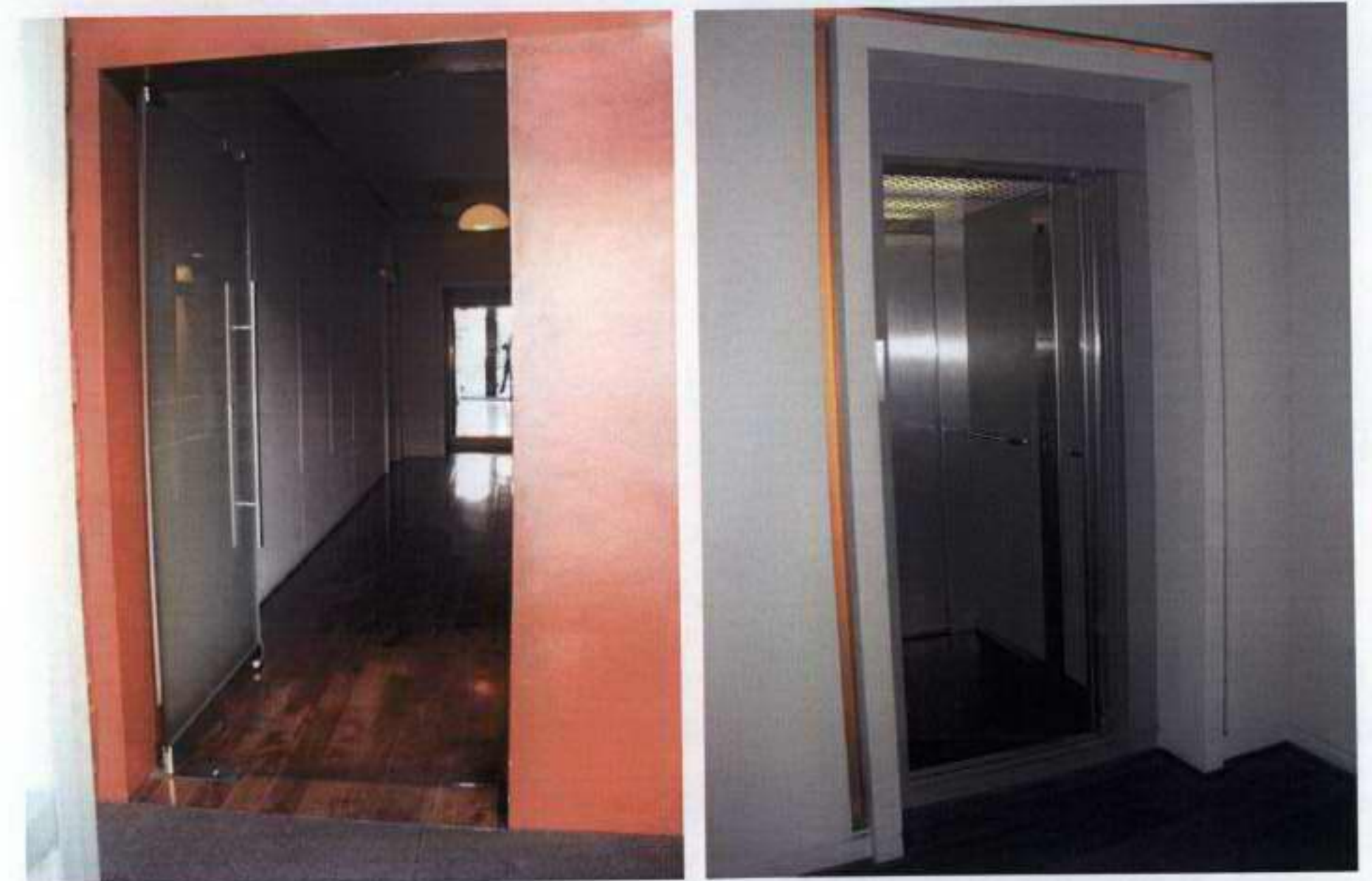
Fig. 7 Photographs showing the level thresholds at the main entrance and lift at 55 Holmes Road.
