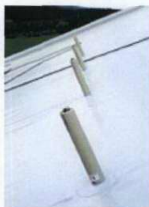
Screwing to steel supports
