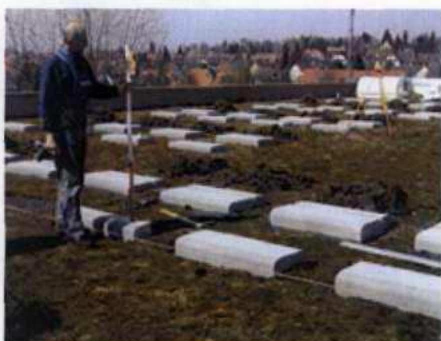
Solid concrete foundations, close-butted or linear
