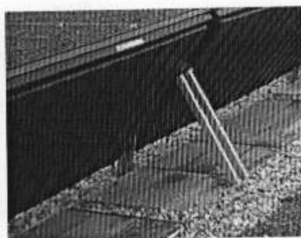
Loading of the supports by concrete slabs or gravel
