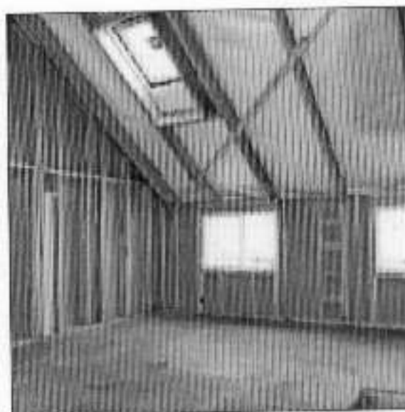
Roofs constructed from Masonite Beams offer the immediate benefit of extra roof space. This example shows the rafters at 1200mm centres – in contrast to the normal 600mm spacing in conventional fink truss roofs.
