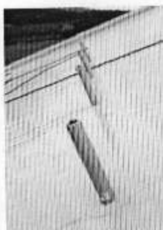
Screwing to steel supports
