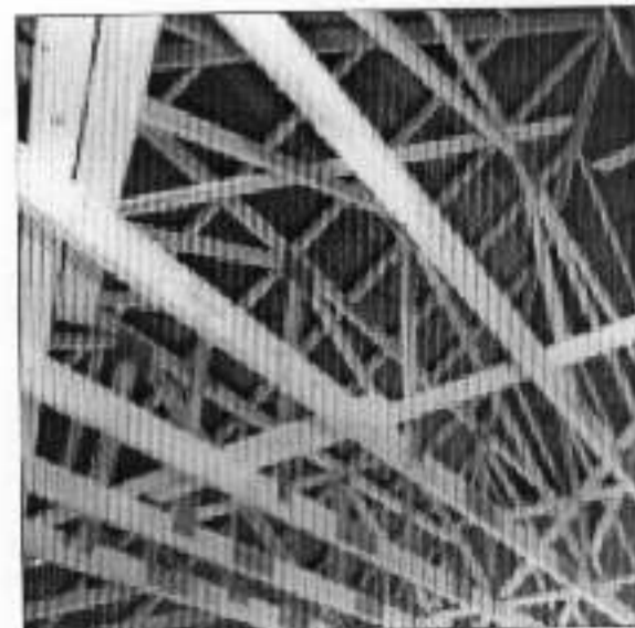
A typical fink truss roof construction, featuring a mass of cross ties and struts taking up valuable space that a Masonite roof would transform into an additional 'Room In the Roof'.
