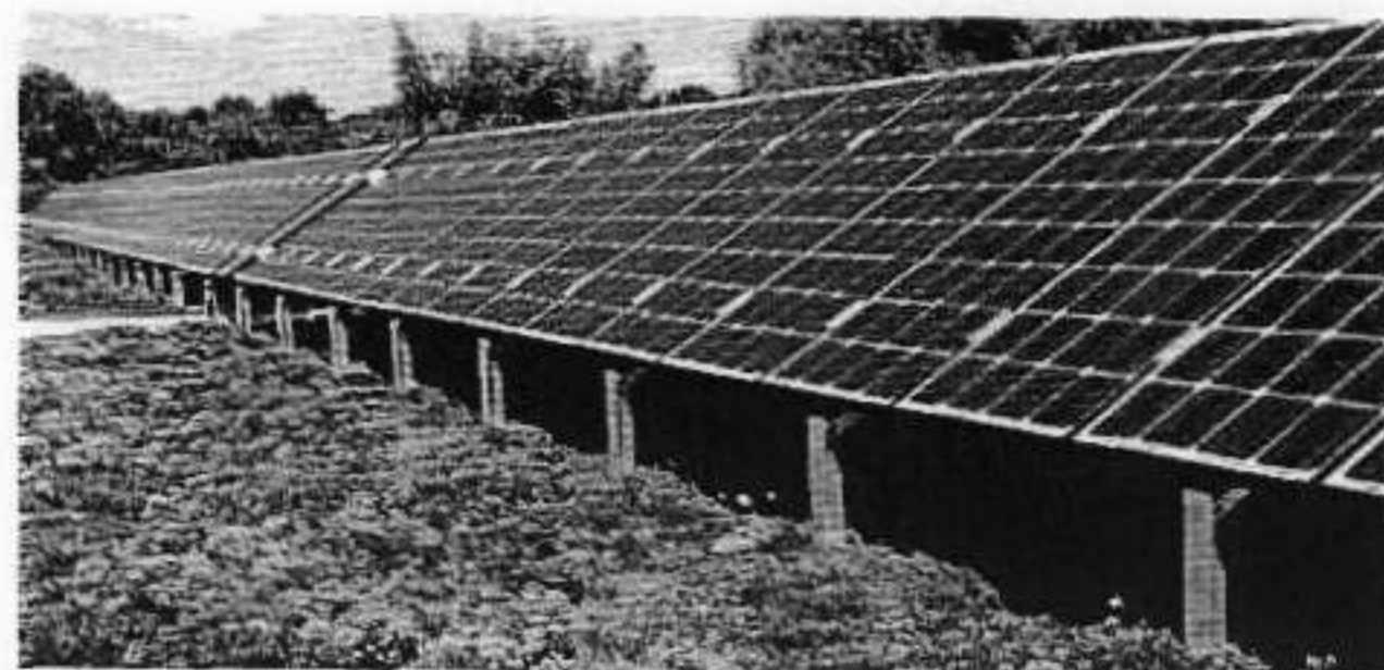
Fig. 23 Photograph of a hybrid solar panel, grass roof system in operation.
