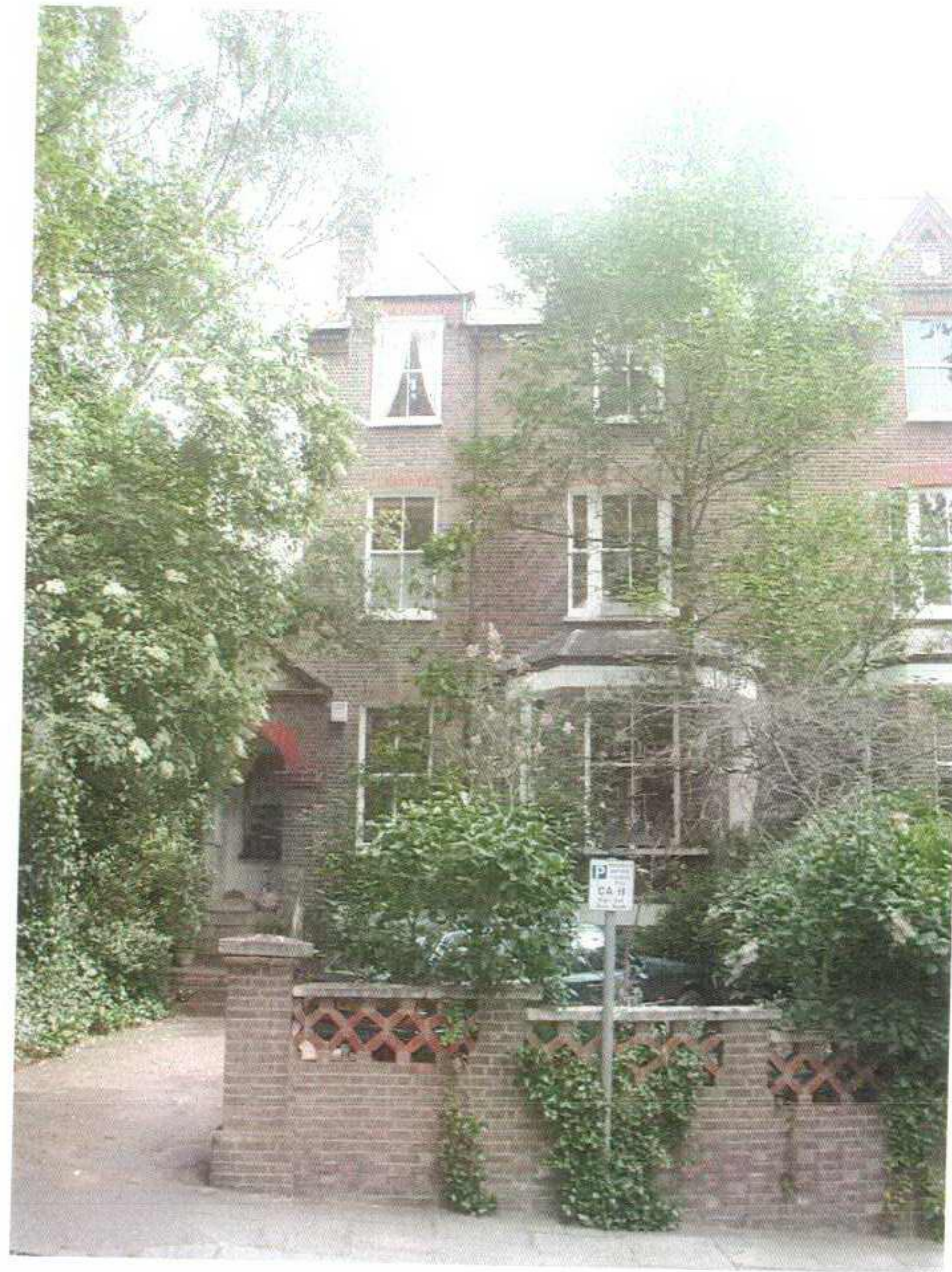
Photograph 7 - 22 Christchurch Hill - Front Elevation.
