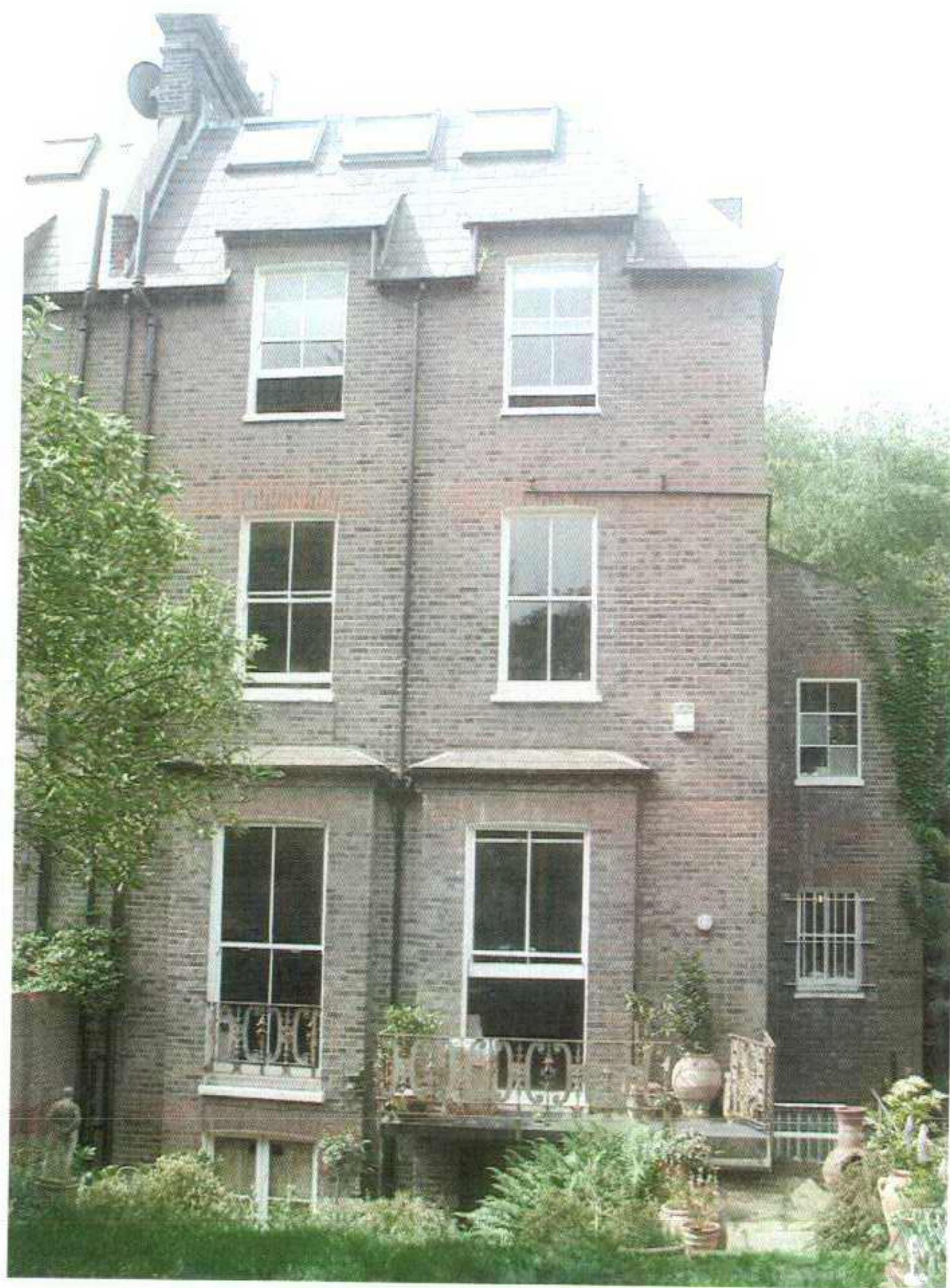
Photograph 5 - 22 Christchurch Hill - Rear Elevation.
