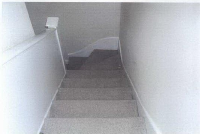
2ND FLOOR LANDING - DOWN
