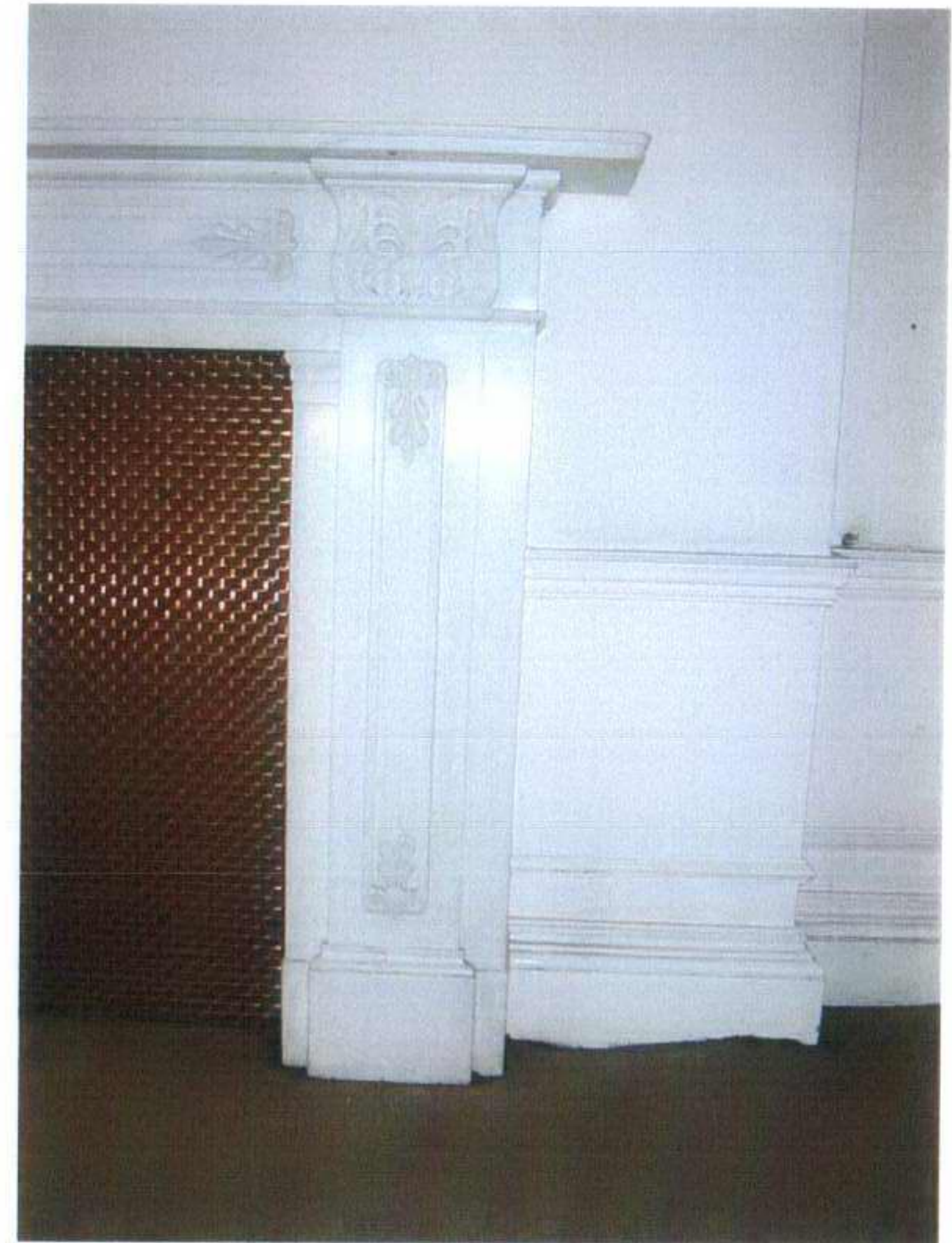
22 Existing fireplace first floor front room No.52
