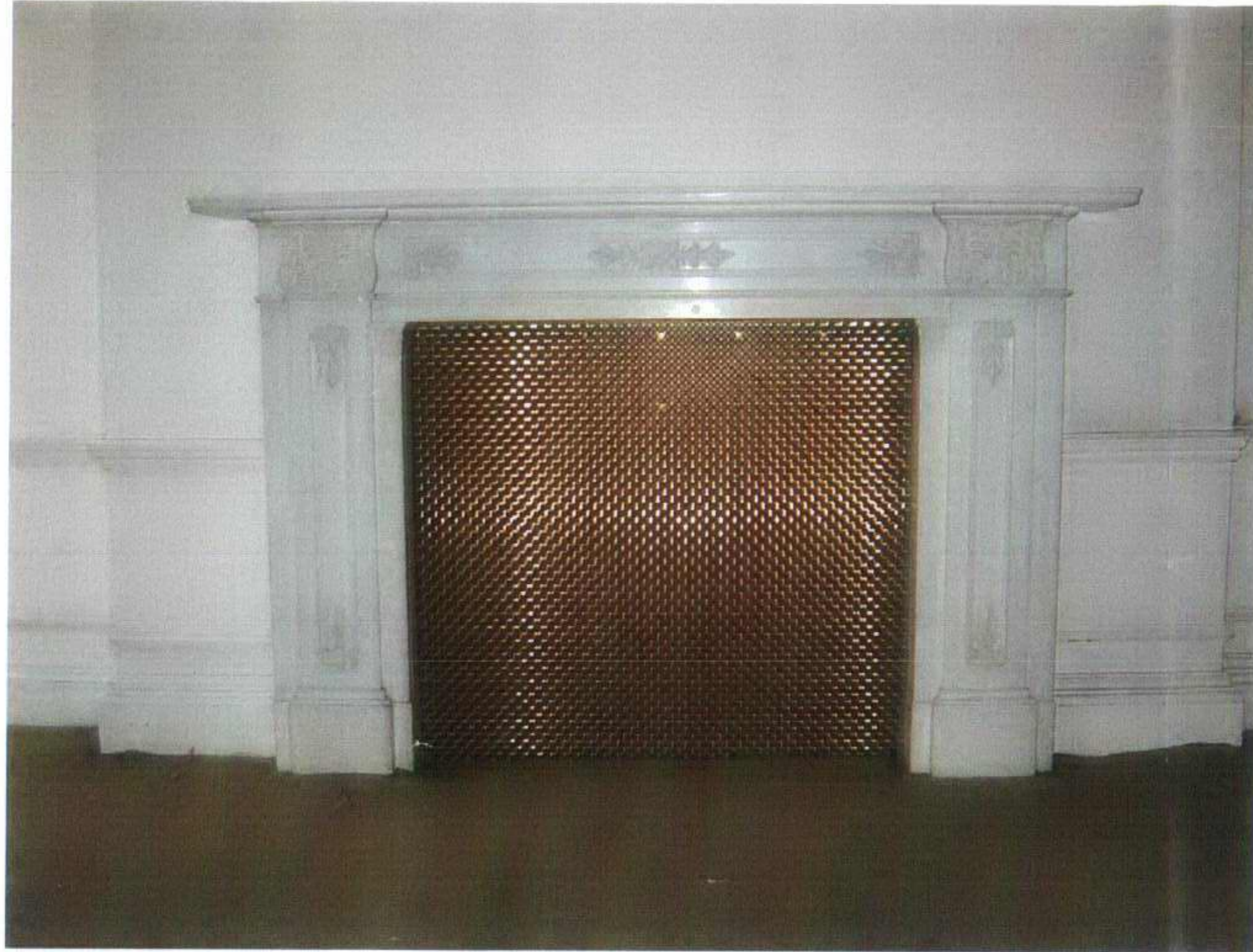
21 Existing fireplace first floor front room No.52
